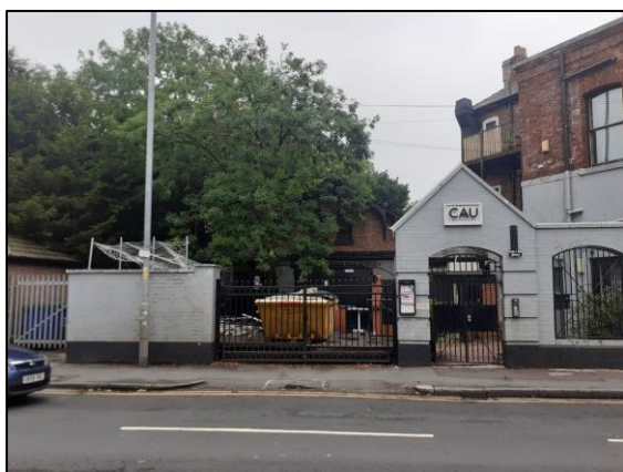
Figure 4: View looking across Barlow Moor Road to the existing rear outdoor seating area.
