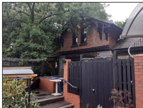
Figure 5: View of existing rear outdoor seating area towards coach house building.
