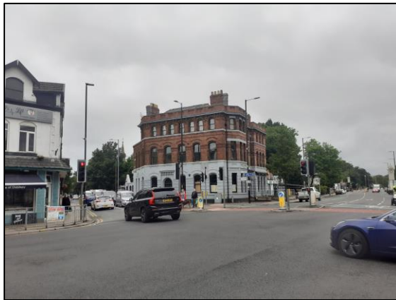
Figure 2: View of 700 Wilmslow Road from the south.
