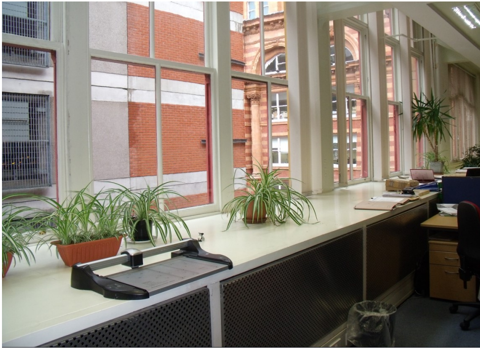
Figure 7: Original inspection/cutting bench encased with the boxing out running along the western side of the office. Sash windows also shown in connection to actuator installation. (Photograph by HE)
