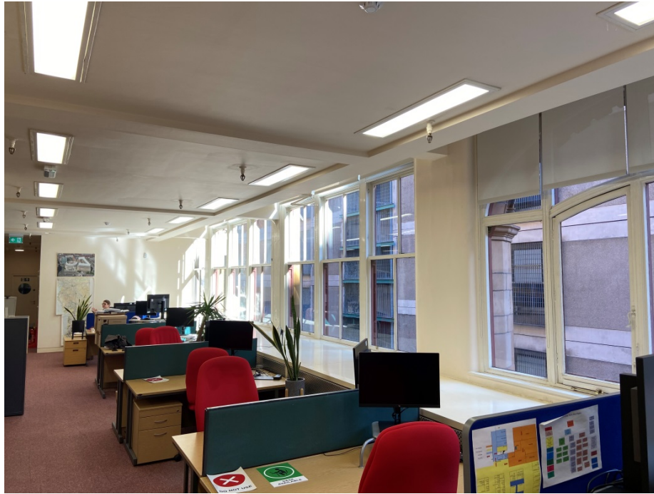
Figure 9 –Boxing out detail over heating system and sash windows visible (Photograph by HE)
