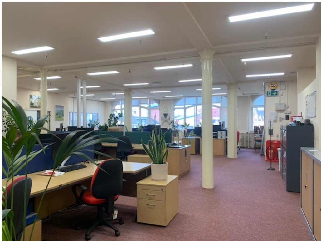
Figure 6 – Internal view looking south showing the different style in columns throughout the floor (Photograph by HE)
