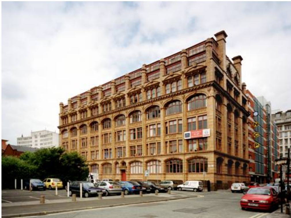
Figure 1 - External view of western and southern facades of Canada House (AA022681 – English Heritage Archives).
