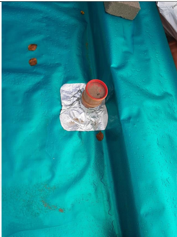
Photograph 8: Validation of Gas Membrane Installation
