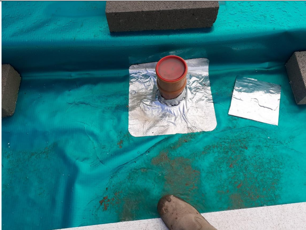
Photograph 5: Validation of Gas Membrane Installation
