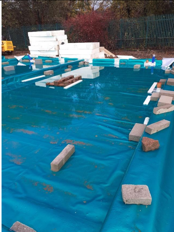
Photograph 7: Validation of Gas Membrane Installation
