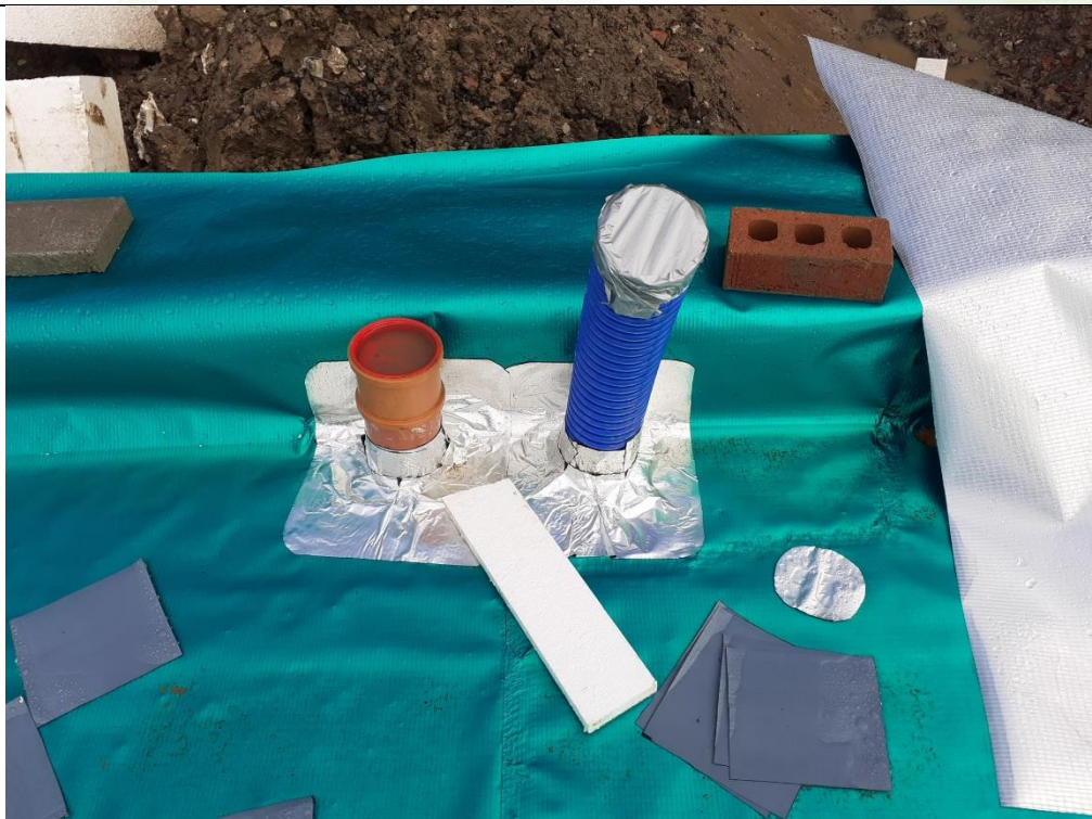
Photograph 6: Validation of Gas Membrane Installation
