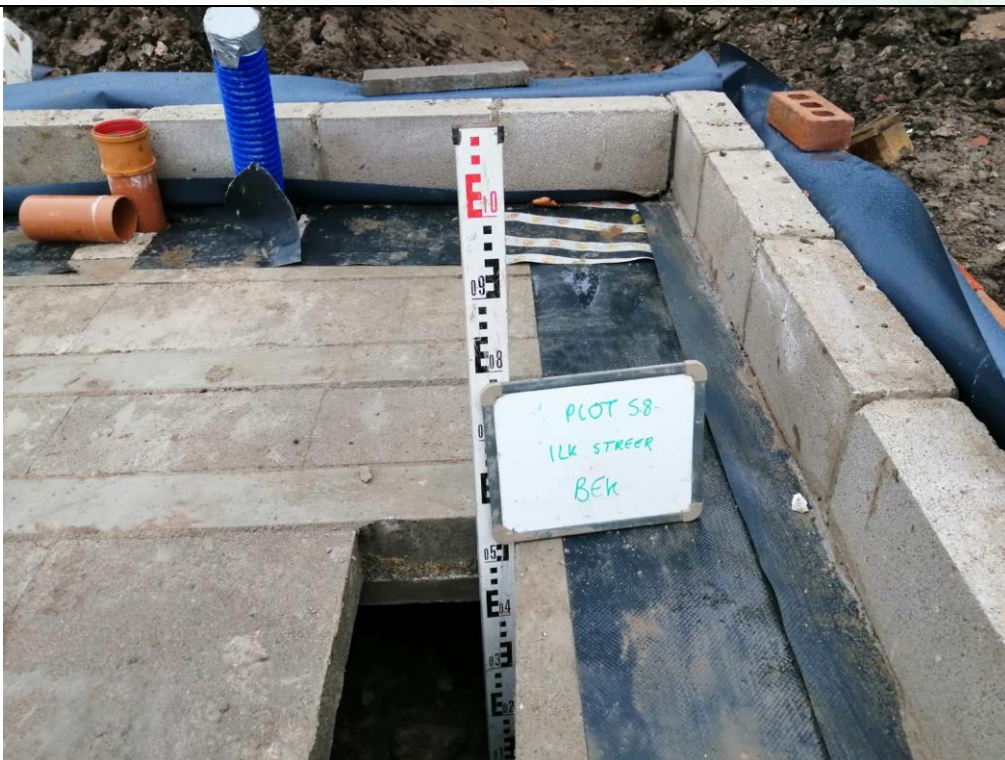
Photograph 4: Validation of Sub-Floor Void Space (min 150 mm)
