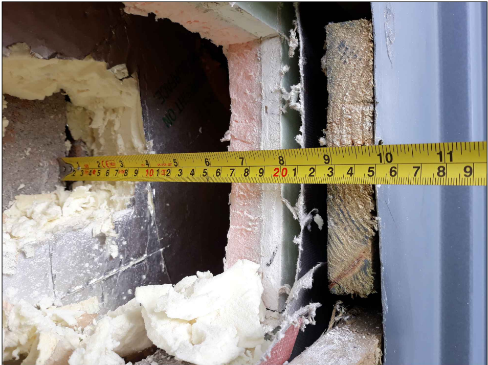
Photograph of existing zinc cladding build-up
