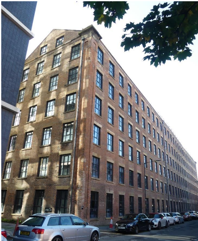
Figure 4.2: The Chapeltown Street elevation of the Crusader Works viewed from the north
