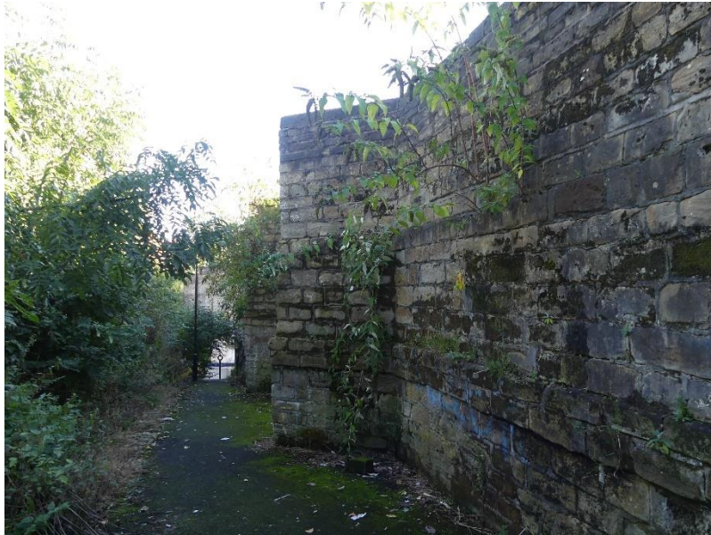
Figure 4.11: The impressive row of triangular buttresses to the northern elevation
