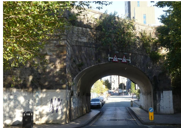
Figure 4.10: The southern side of the skewed arch
