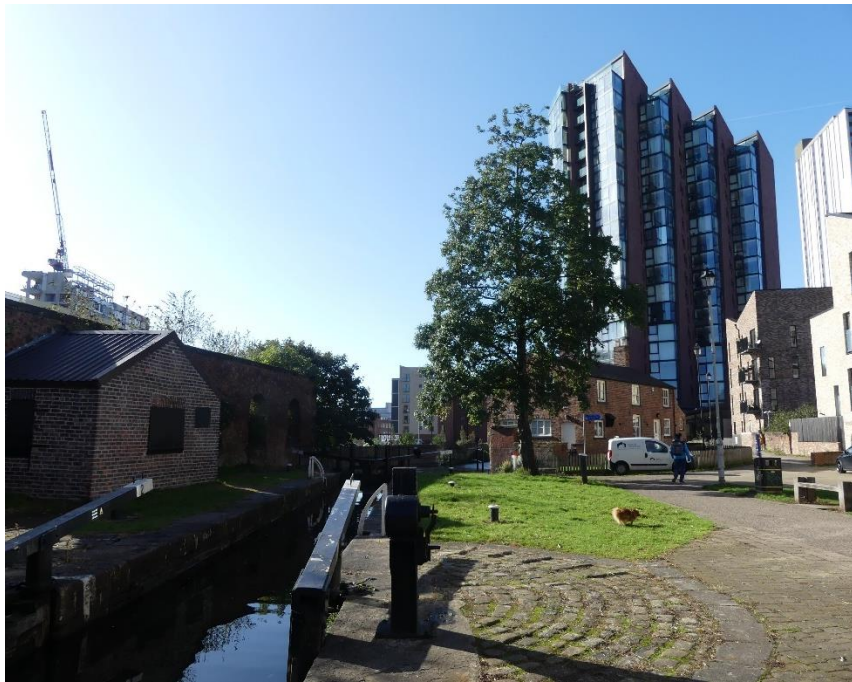
Figure 4.22: Tall-medium rise development in the backdrop to the Lock Keeper's Cottage and Lock No. 2
