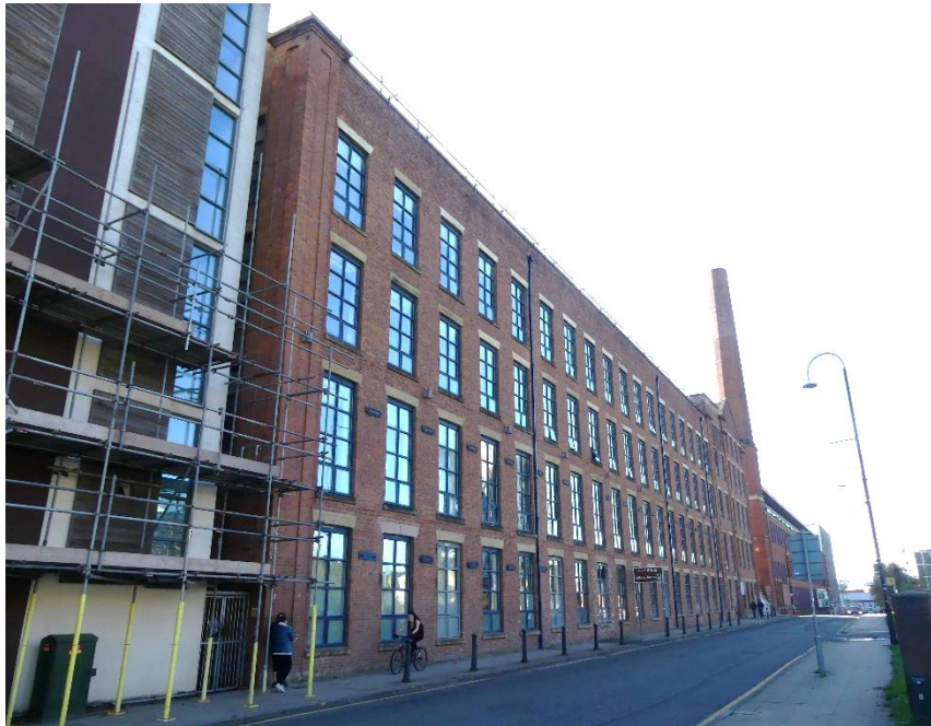
Figure 4.31: The principal, western, elevation to Vulcan Works
