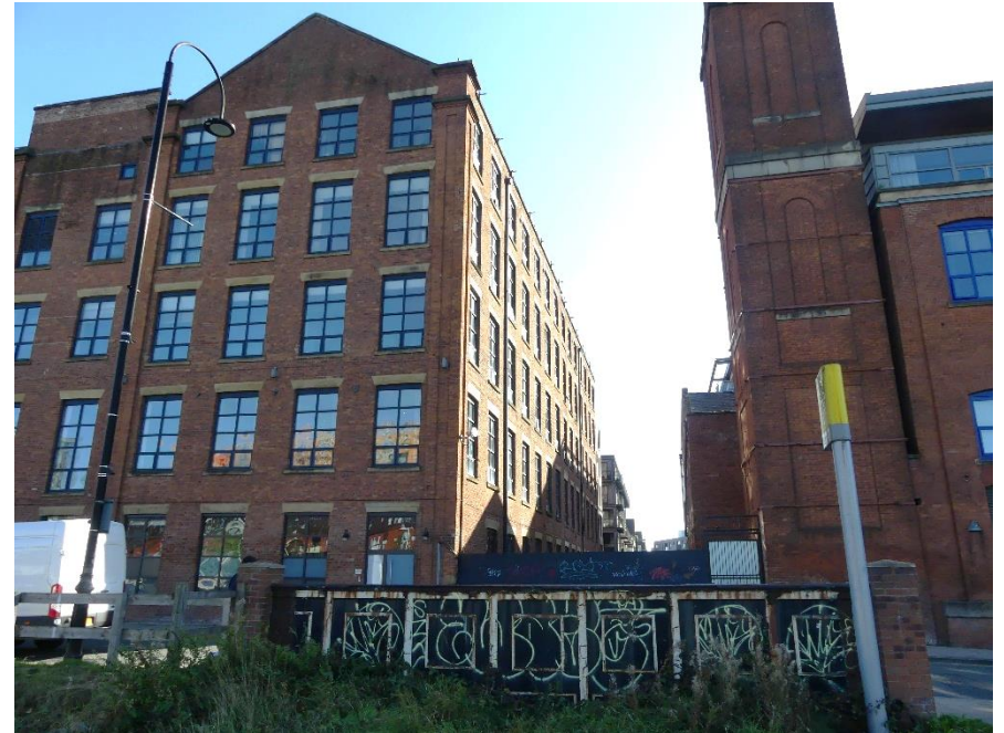
Figure 4.32: The southern elevation facing the former the branch canal
