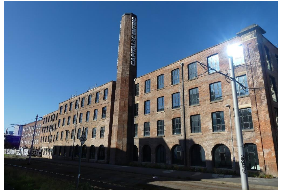
Figure 4.5: The south-eastern elevation
