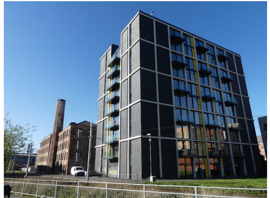
Figure 4.7: Crusader Works and Phoenix Apartments from the north-eastern end of Longacre Street
