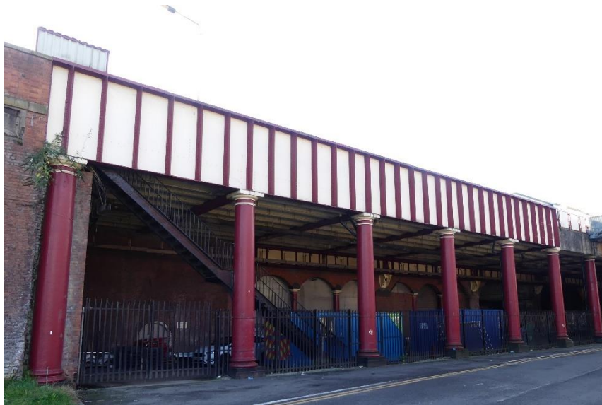
Figure 4.14: The undercroft viewed from Sheffield Street
