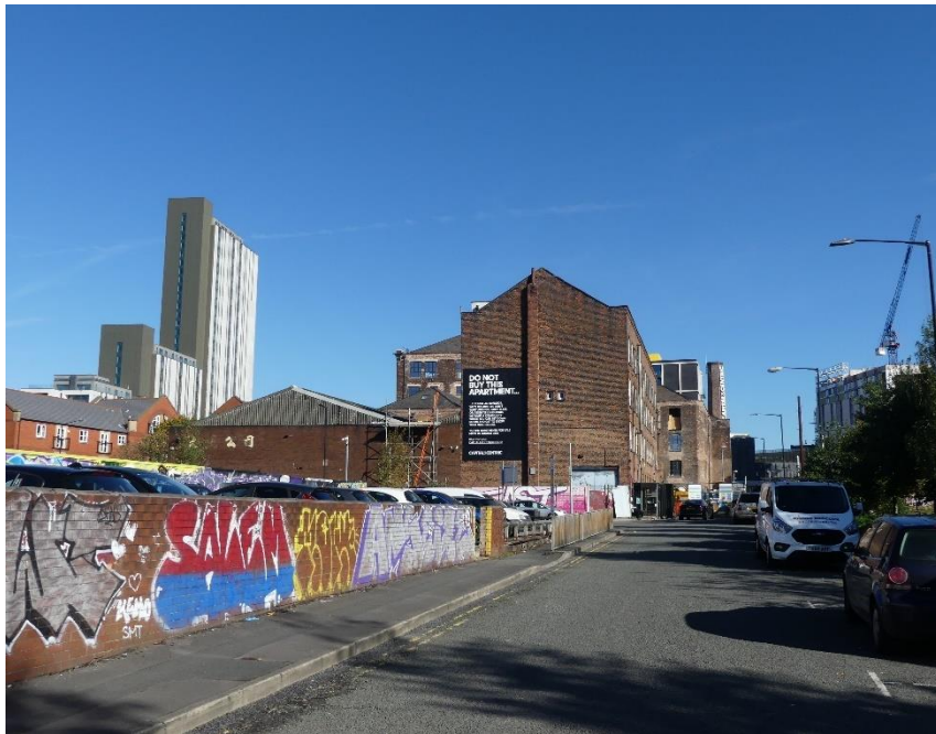
Figure 4.8: The view towards Crusader Works from the south-western part of Longacre Street
