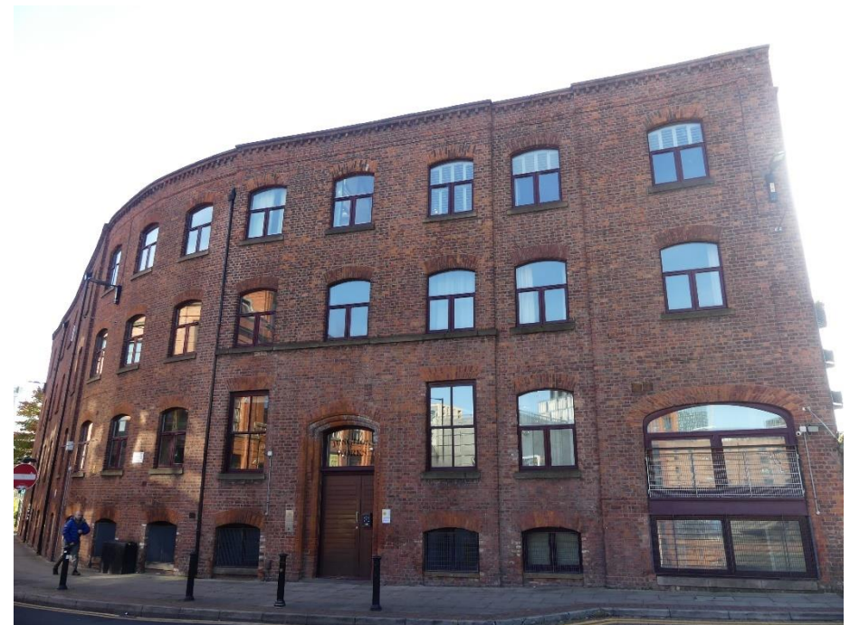
Figure 4.24: The Ducie Street elevation of Junction Works
