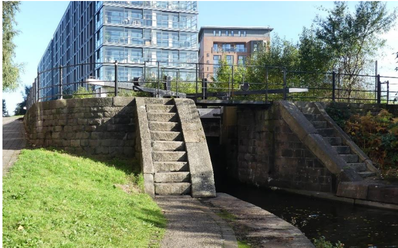
Figure 4.20: The curved staircases flanking the lower end of Lock No. 3
