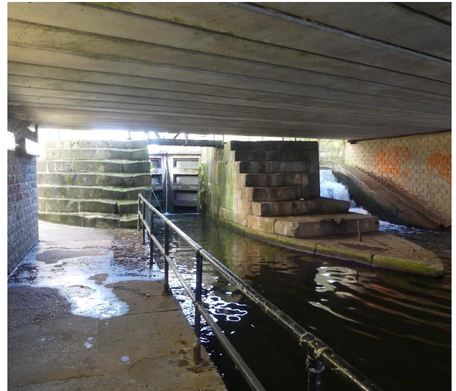
Figure 4.19: The stepped structure of the lock and overflow channel of Lock No. 1 from under Great Ancoats Street
