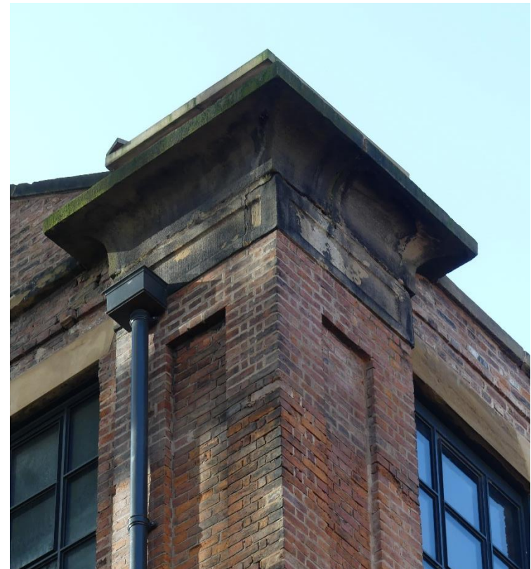
Figure 4.3: Corner detail of the pilaster and capital
