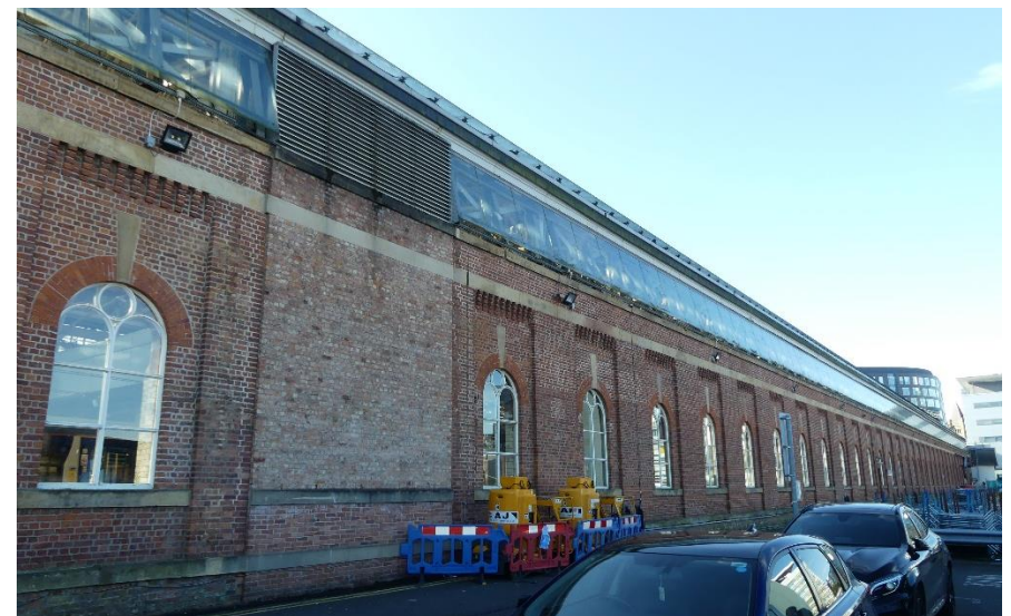
Figure 4.13: The northern elevation of the train shed
