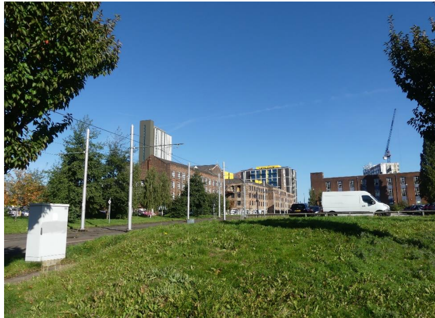
Figure 4.6: The view northwards towards Crusader Works from Sheffield Street
