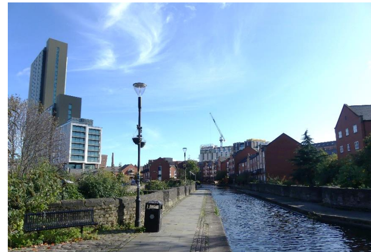
Figure 4.12: The view north-east across the aqueduct
