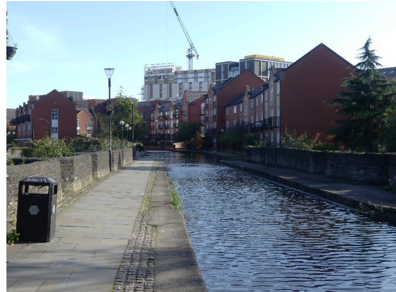
Figure 4.30: The top of the Phoenix apartment development is just visible in the view north from Store Street Aqueduct
