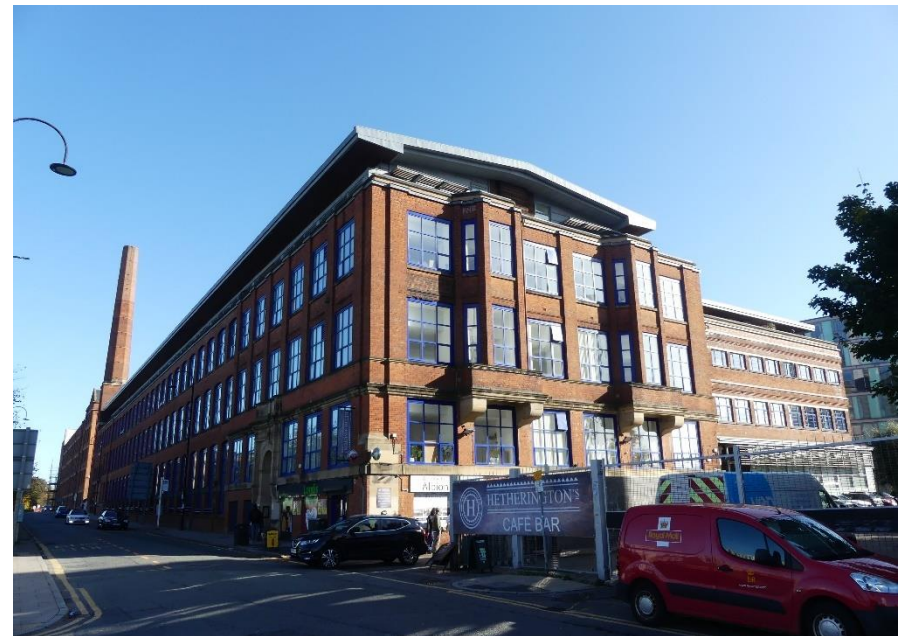
Figure 4.16: The oriel windows of the southern elevation and the western elevation leading to Vulcan Works
