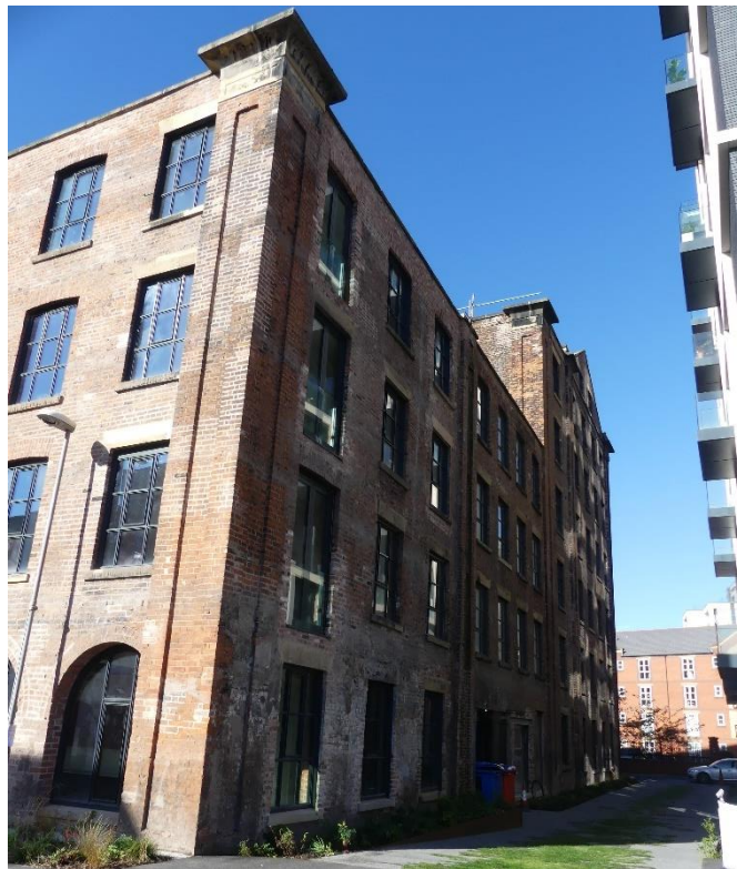
Figure 4.4: The north-eastern elevation to Fair Street
