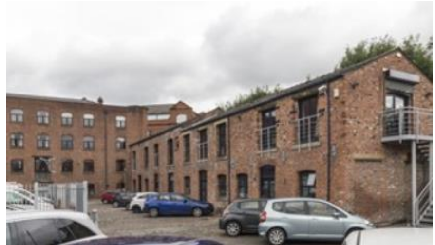
Figure 4.26: The former Stable Block located to the rear of Junction Works
