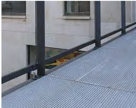
P9 - STEEL DECKING
