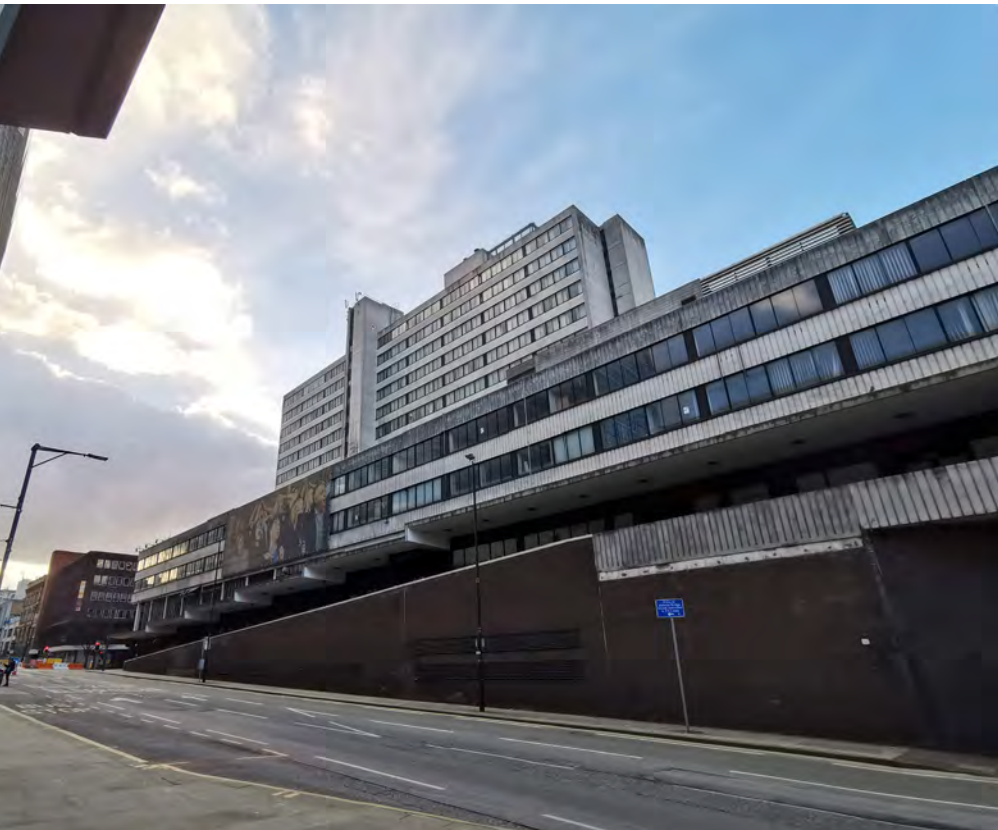
1. View of existing inactive frontage along Deansgate
