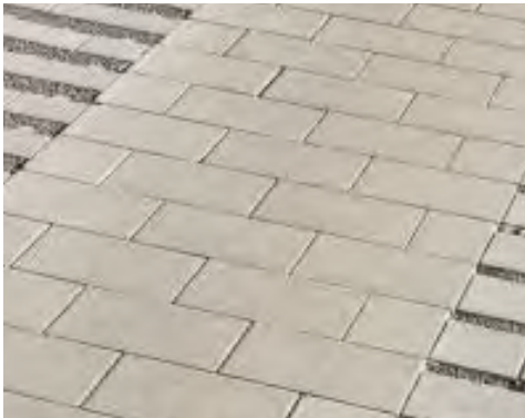
P7 - CONCRETE PAVING (PERMEABLE)
