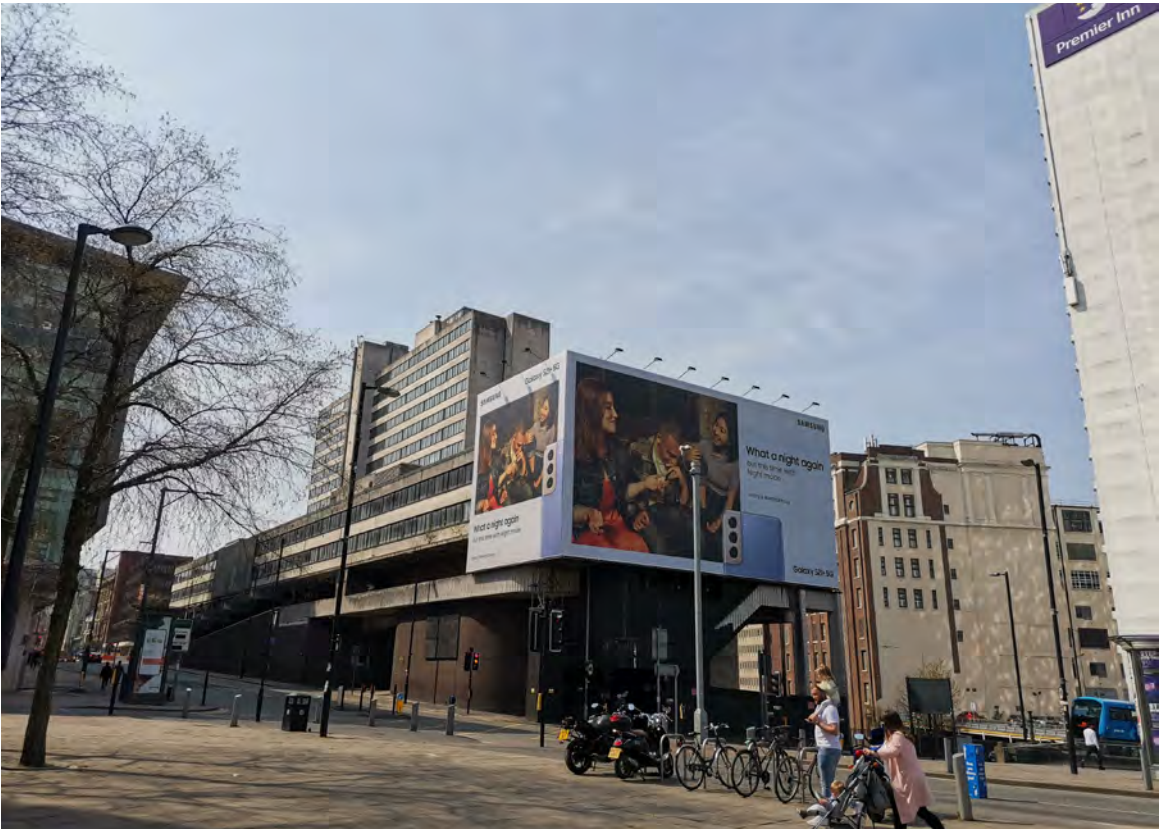
2. Existing view from Medieval Quarter down Deansgate
