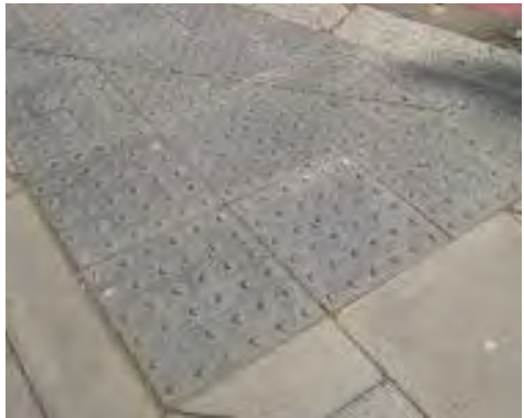
P6 - TACTILE BLISTER PAVING
