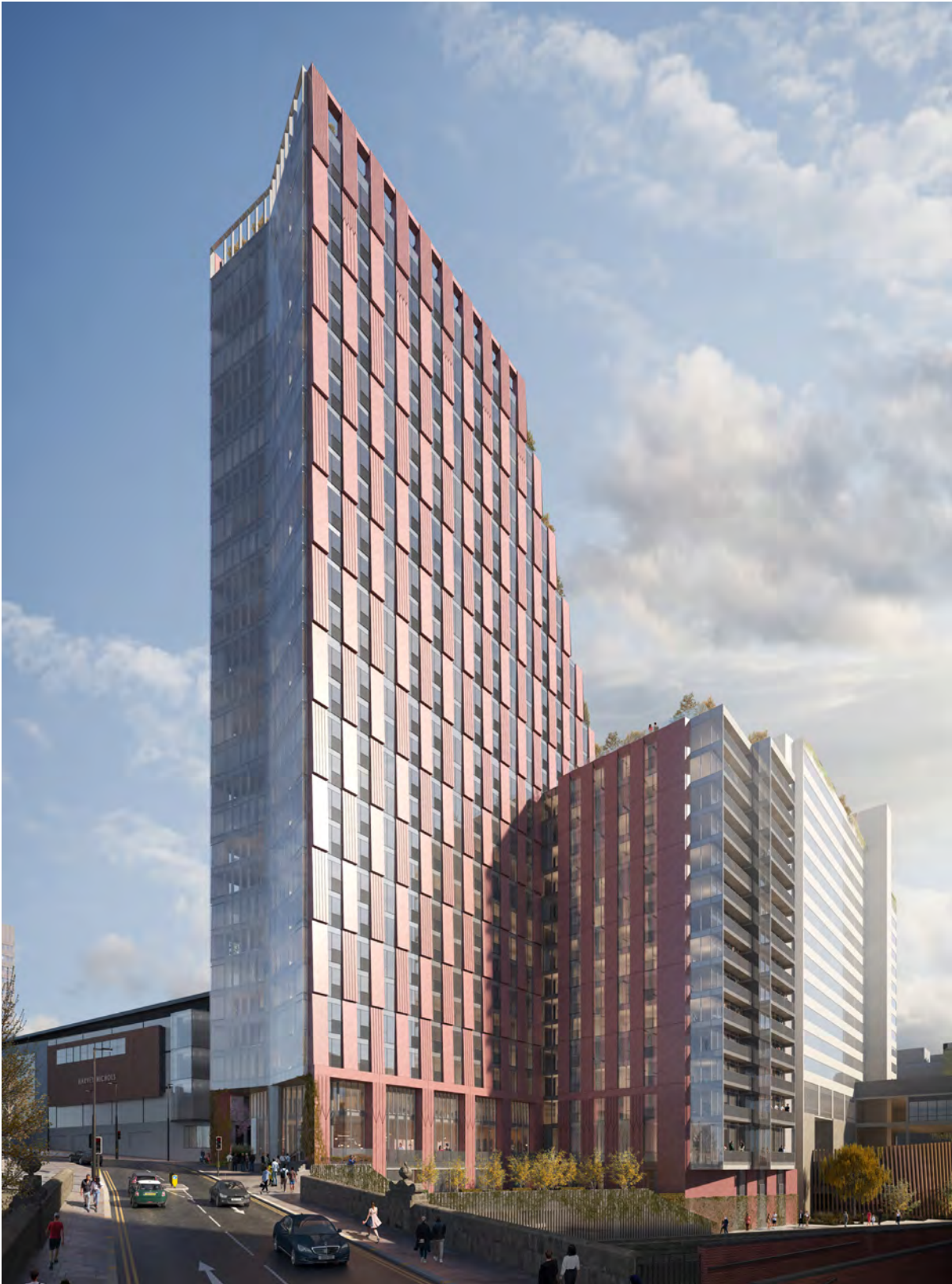
2. Dusk view from Victoria Bridge Street
