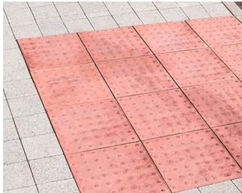
P5 - TACTILE BLISTER PAVING
