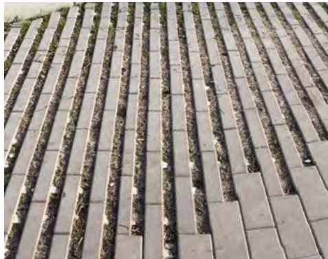
P8 -GRAVEL GAP PAVING (PERMEABLE)
