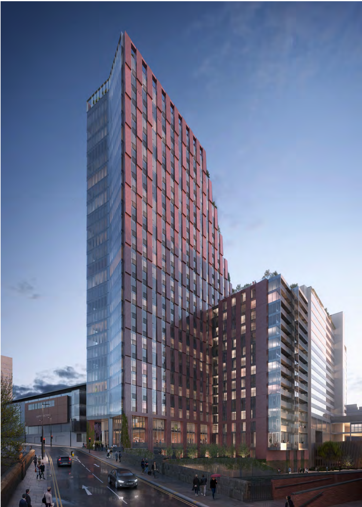
3. Dusk view from Victoria Bridge Street
