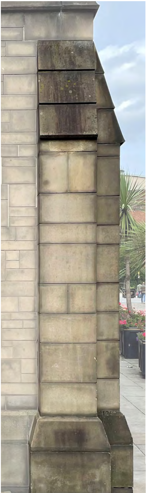
Stone Shingle Detailing
