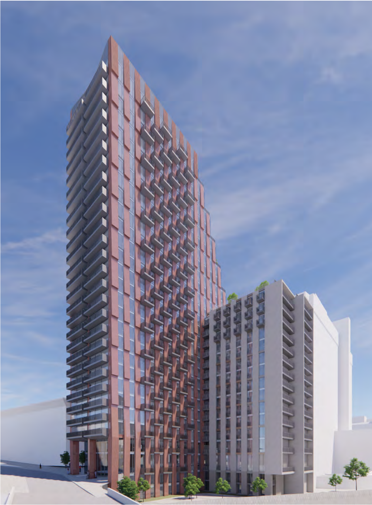
2. View from Victoria Bridge Street
