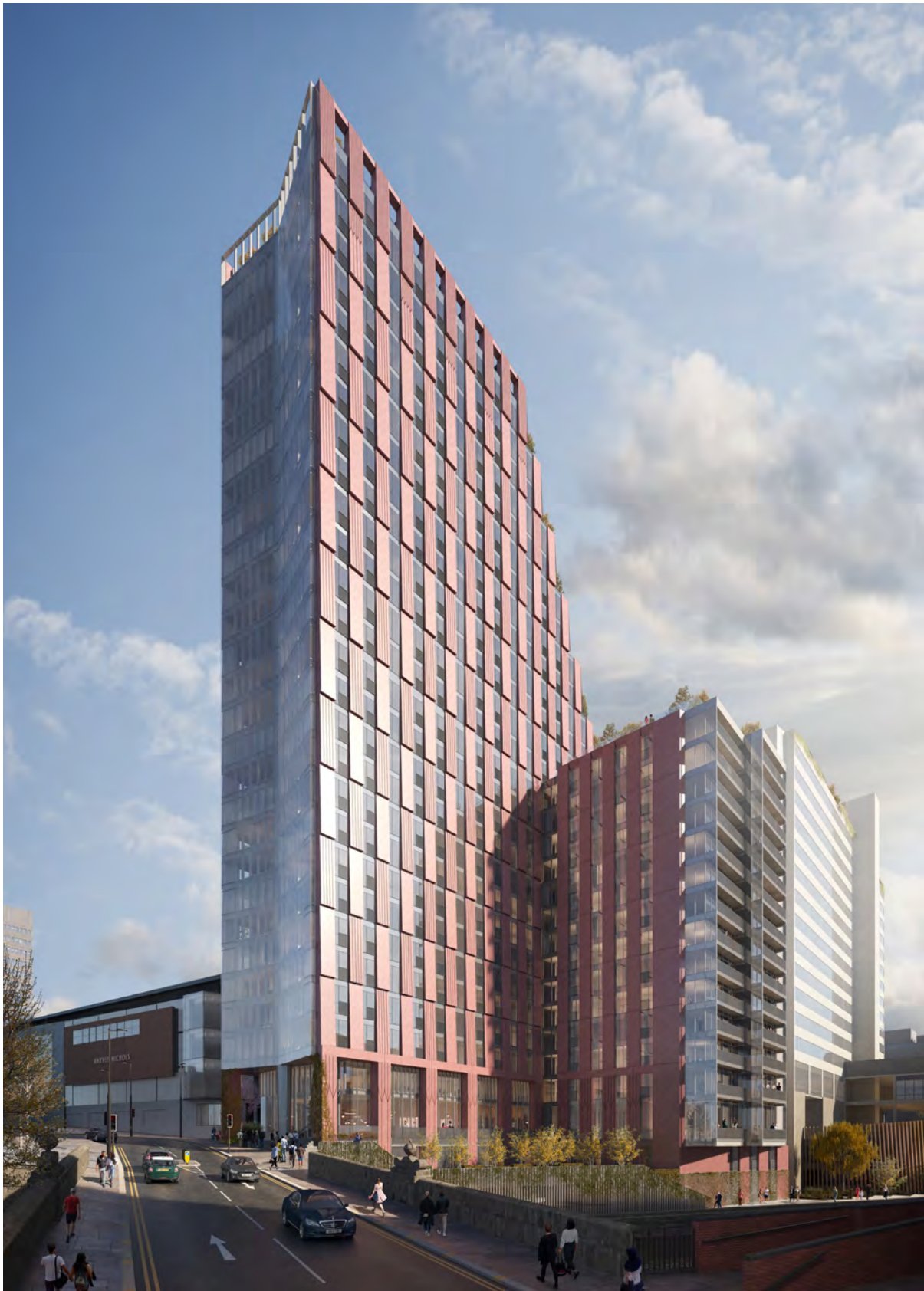
3. View from Victoria Bridge Street
