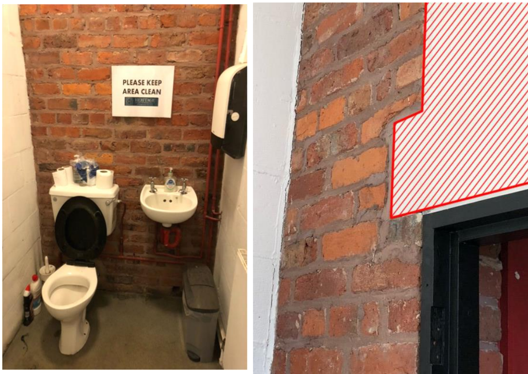
Figure 1. (left) Where existing plumbing fixtures and blockwork walls are removed, localised brick repairs are to be undertaken to match the surrounding masonry.
