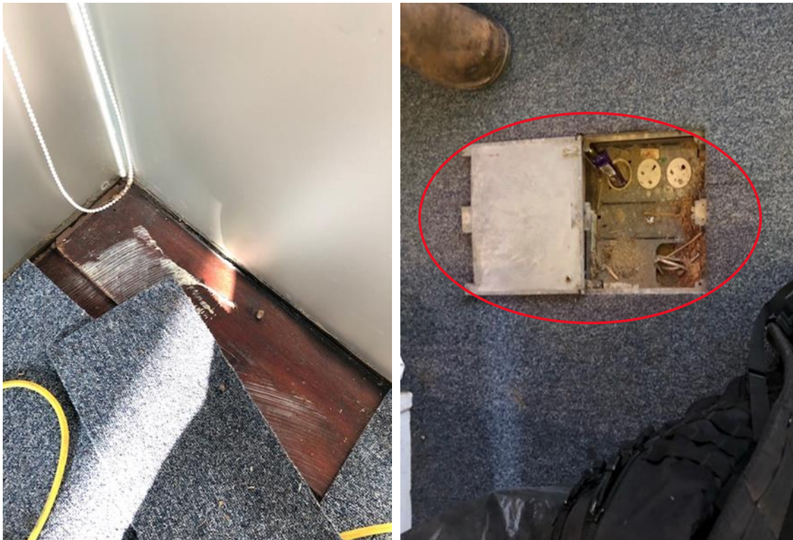
Figure 3. (Left) Carpet tiles to be removed and existing floorboards to be levelled, cleaned and repaired as required, prior to installing new floor finishes. (West classroom)
