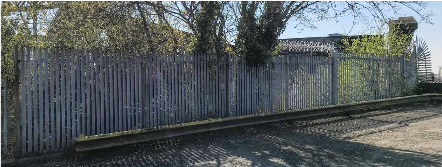
Photo of existing palisade fence and gate
