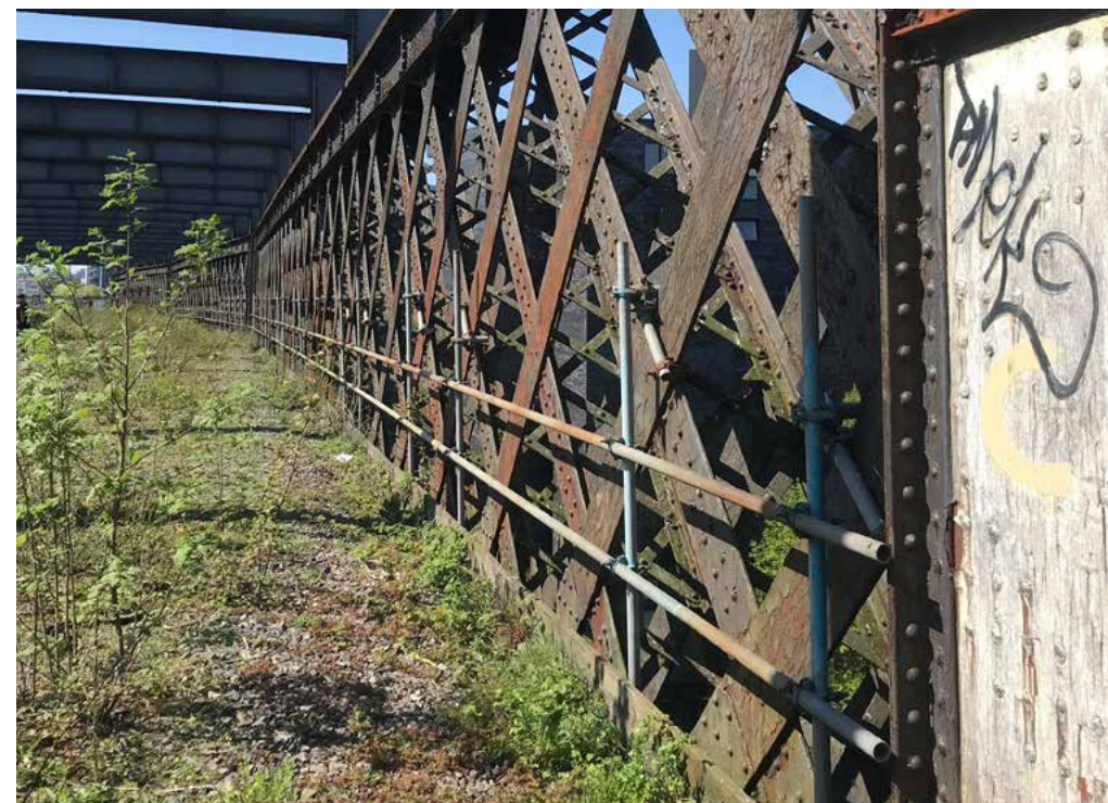
Photo of existing scaffolding poles
