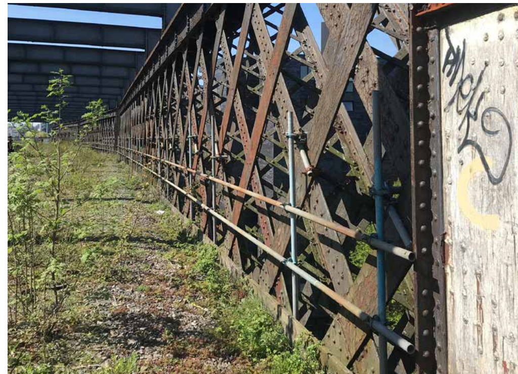
Photo of existing scaffolding poles
