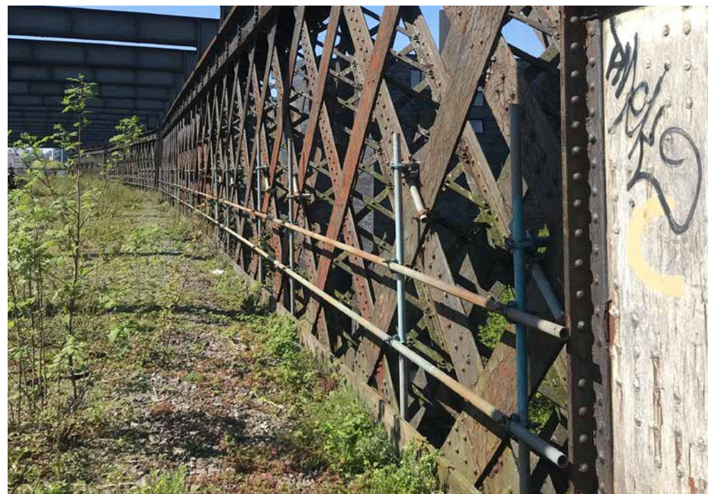
Photo of existing scaffolding poles
