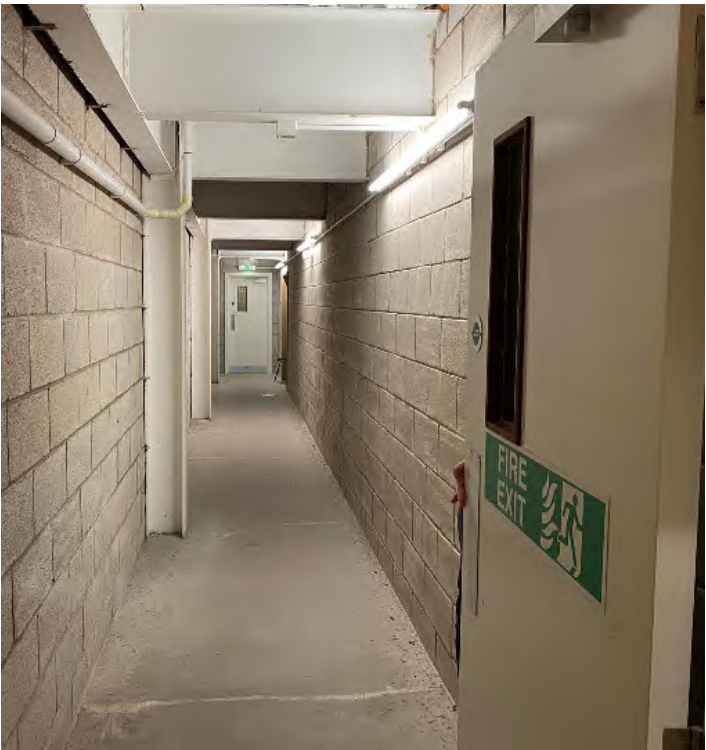
Basement storage area corridor
