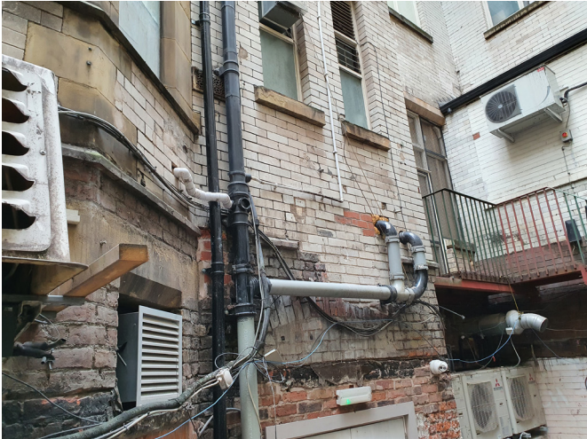
mage 04: Existing Lightwell
