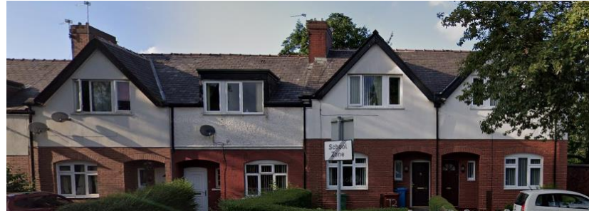
Existing houses along Victoria Avenue
