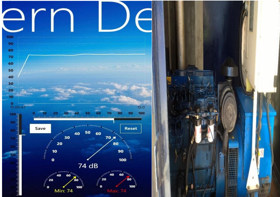
Figure 9.1.5 Generator noise levels uncontained.
