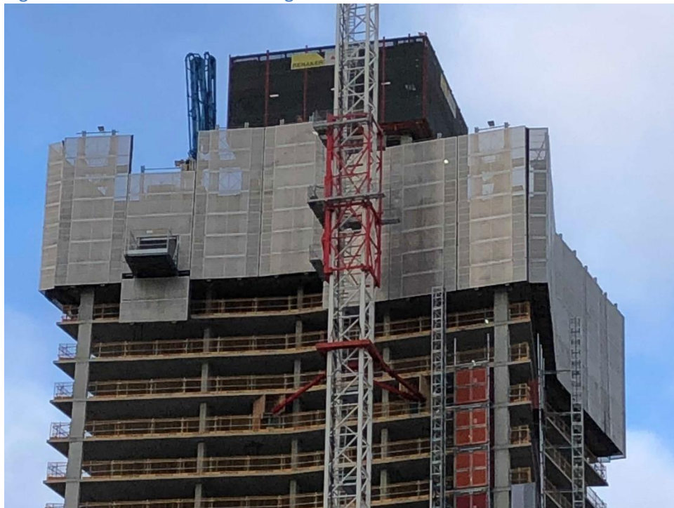
Figure 9.1.1 – Screens surrounding concrete works
