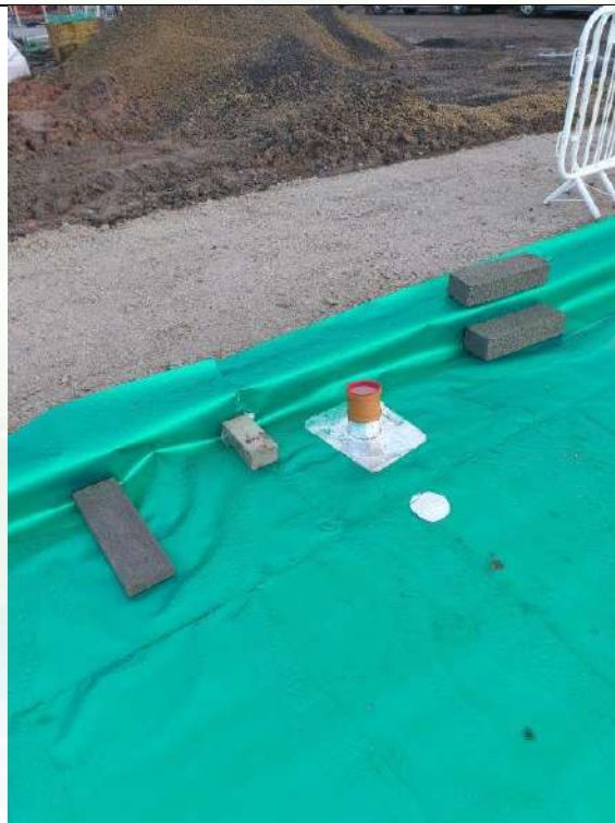
Photograph 8: Validation of Gas Membrane Installation
