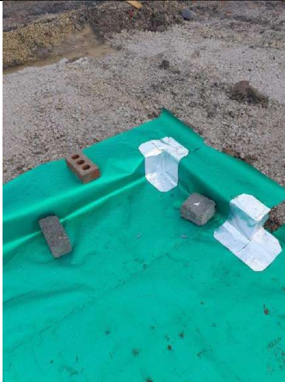
Photograph 5: Validation of Gas Membrane Installation
