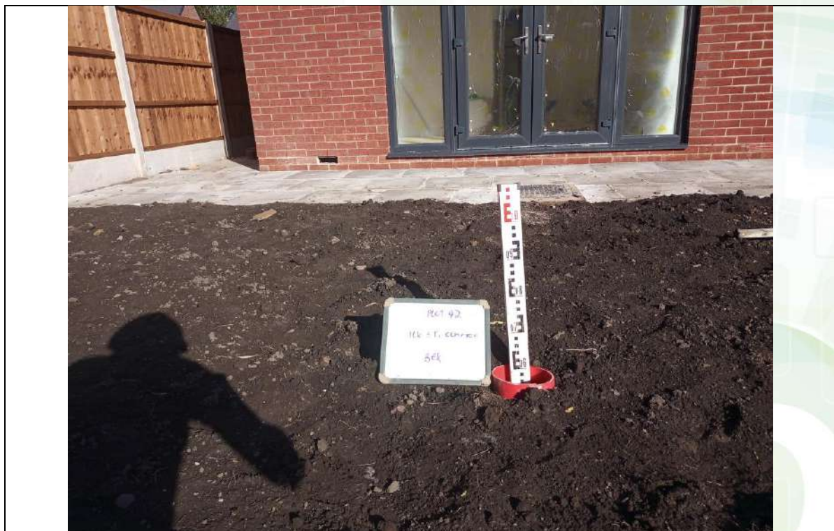
Photograph 2: Validation of Garden Capping Thickness
