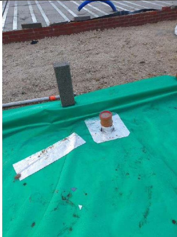
Photograph 7: Validation of Gas Membrane Installation
