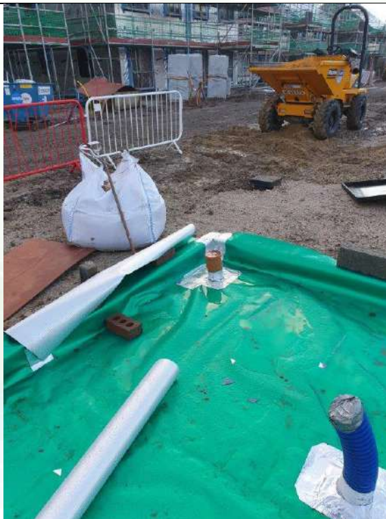
Photograph 6: Validation of Gas Membrane Installation
