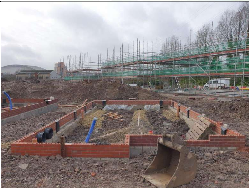
Photograph 4: Validation of Sub-Floor Void Space (min 150 mm)
