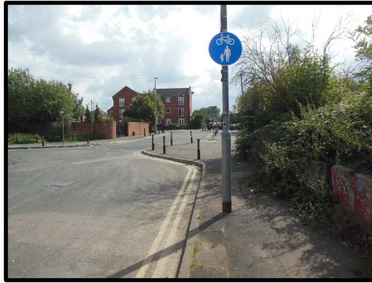
Photo 3-6: Beginning of Shared Footway/Cycleway on approach to MHS entrance
