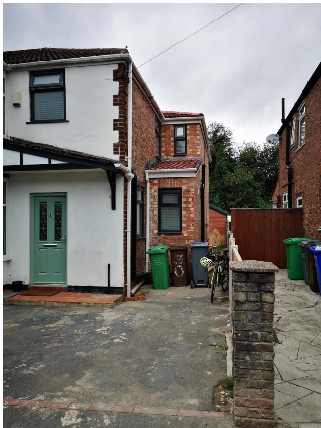
Front view from Saddlewood Avenue with outbuilding visible to the rear
