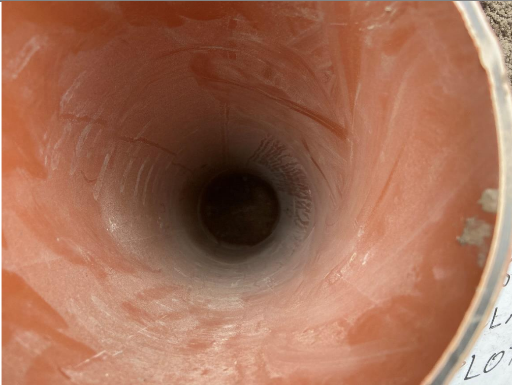
Photograph 3: Validation of Geotextile Membrane
