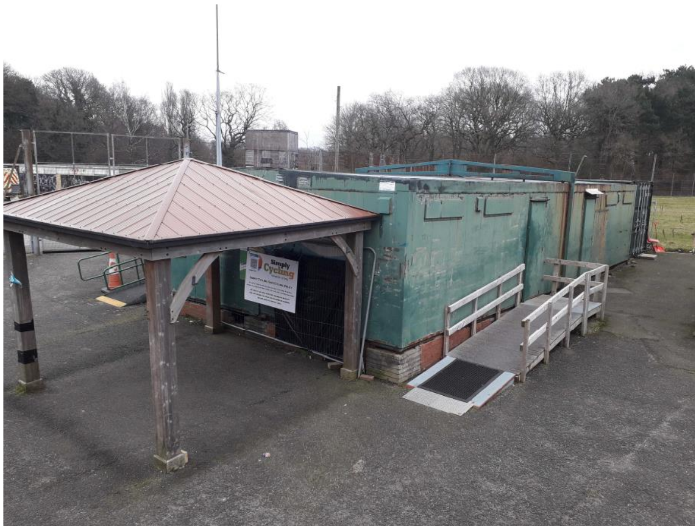
Photograph 1 Existing Changing room facilities – Source: Photograph provided by the applicant
