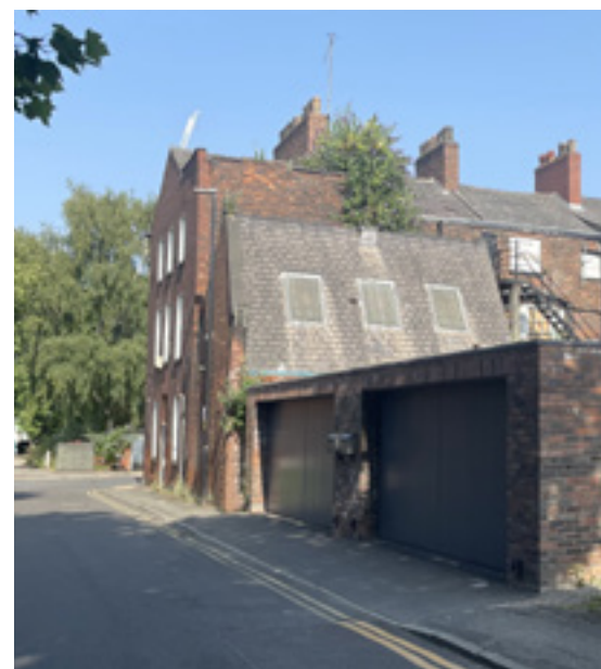
④ 31 Byrom Street Grade II listed mid 19th Century building The former home of the Convent of St. Mary with a small worship space to the rear of the terraced building.
