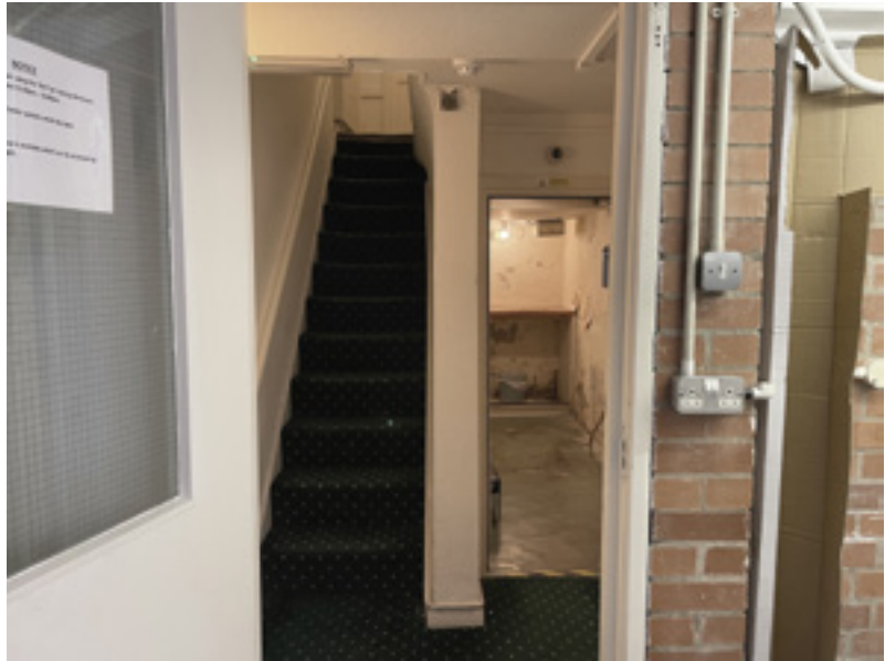
02. View of the staircase from the basement to ground floor
