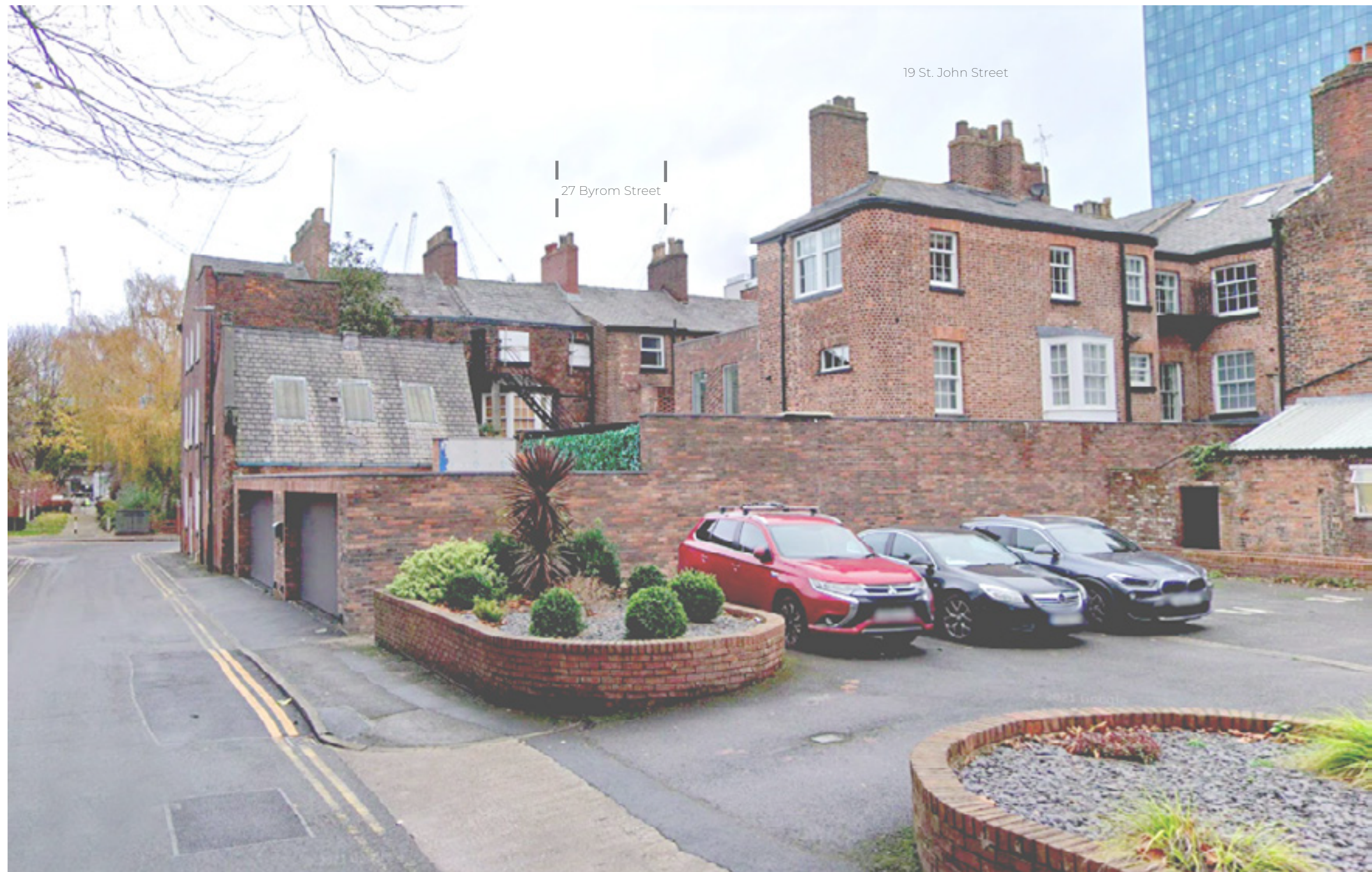
View of the rear elevation of 27 Byrom Street from Camp Street.
