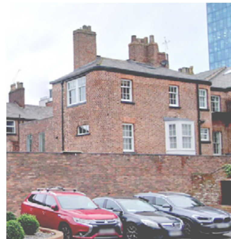
19 St. John street rear extension
