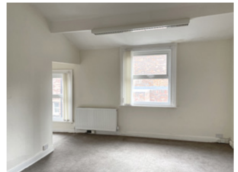
02. Second floor office at the rear of the property. The original line of the rear elevation can be seen the line of structure crossing the room at ceiling level
