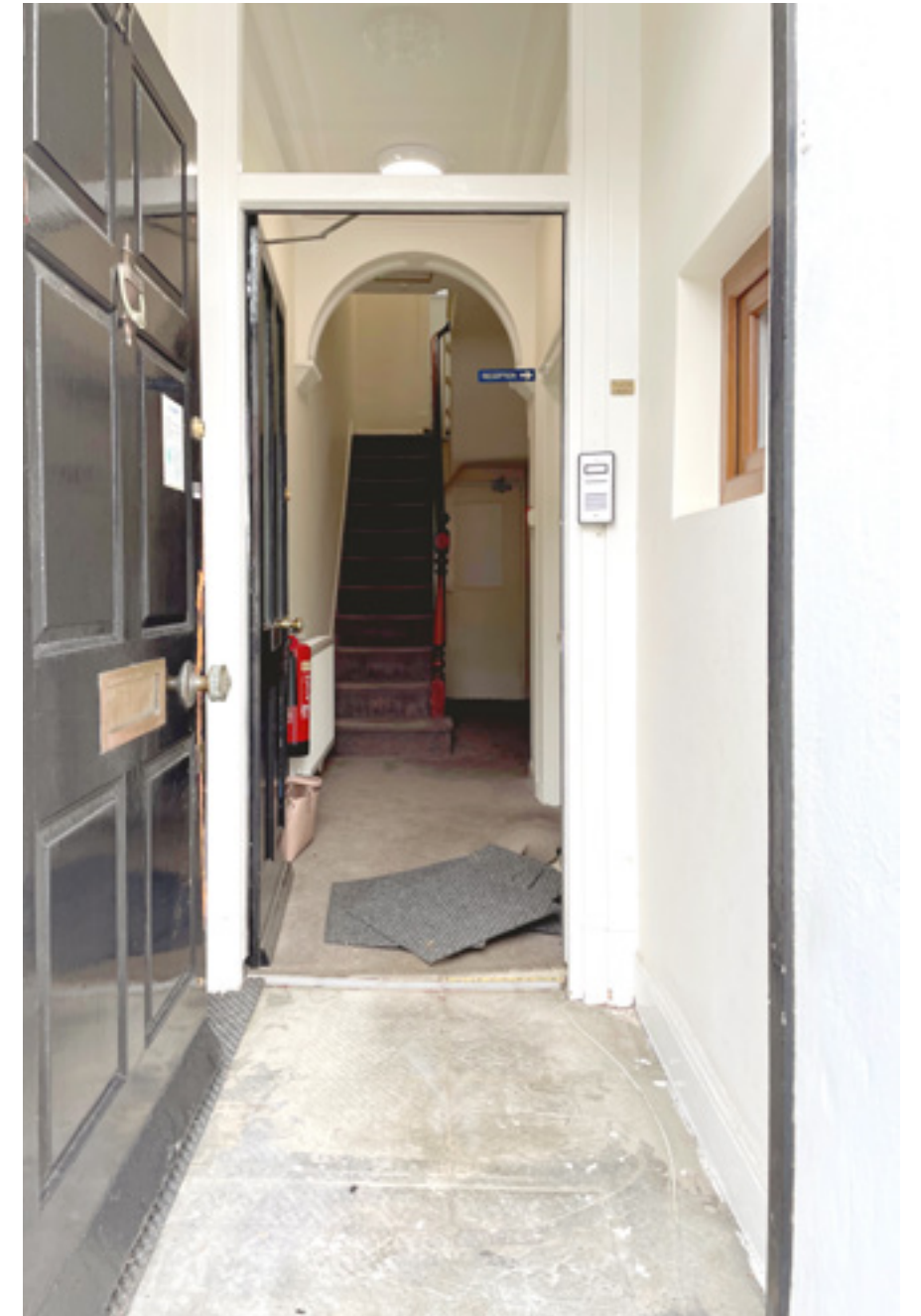
02. View of the entrance hall and staircase
