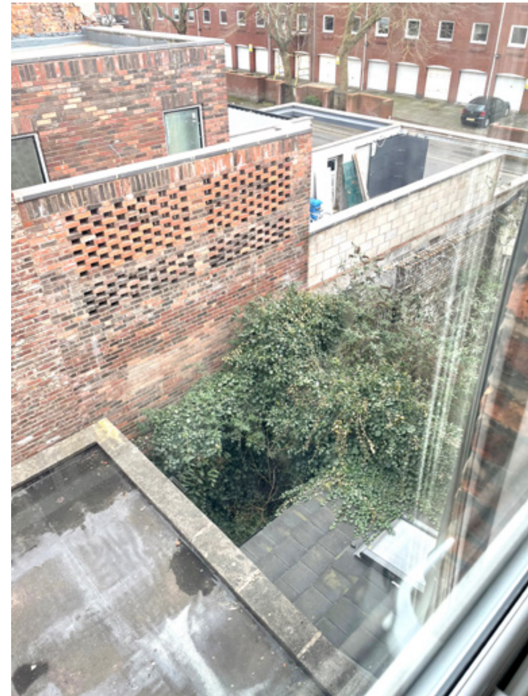
View from the second floor window of 27 Byrom Street Looking at the existing single story flat roof extension to 27 Byrom Street and the empty (overgrown) rear yard of 29 and 31 Byrom Street
