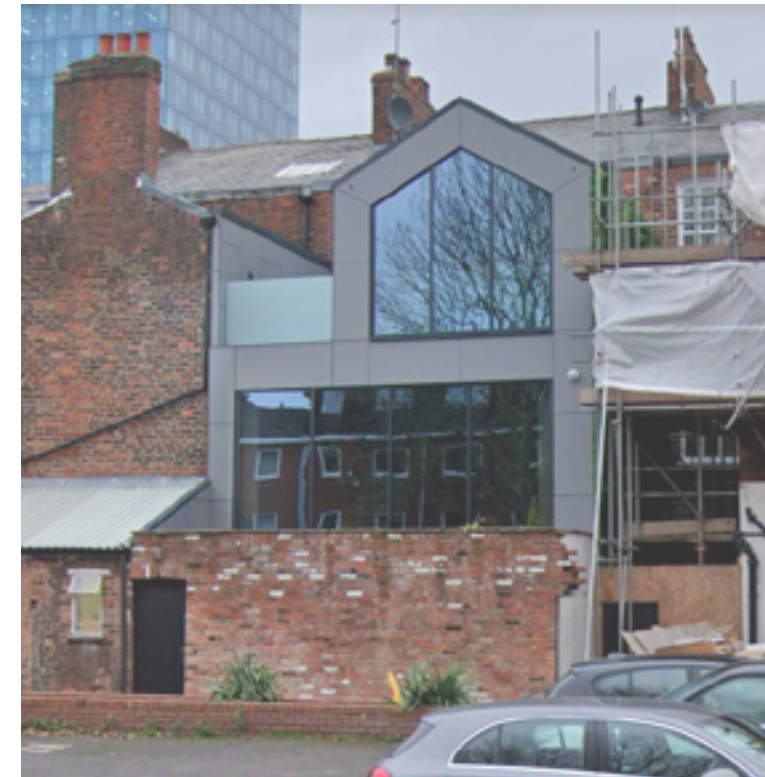
15 St. John street rear extension
