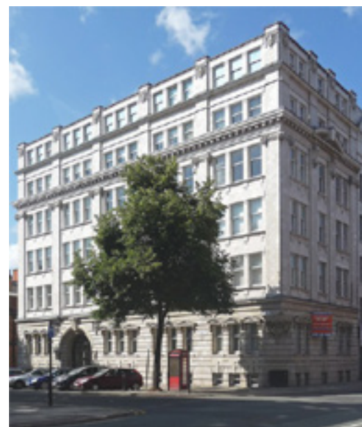
③ 2 St. John Street Grade II listed early 20th Century building A building of significant presence and Portland stone facade on the corner with Deansgate.
