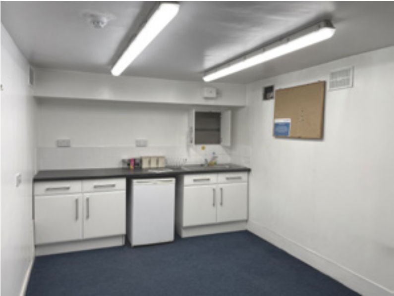
01. View of the existing staff kitchen
