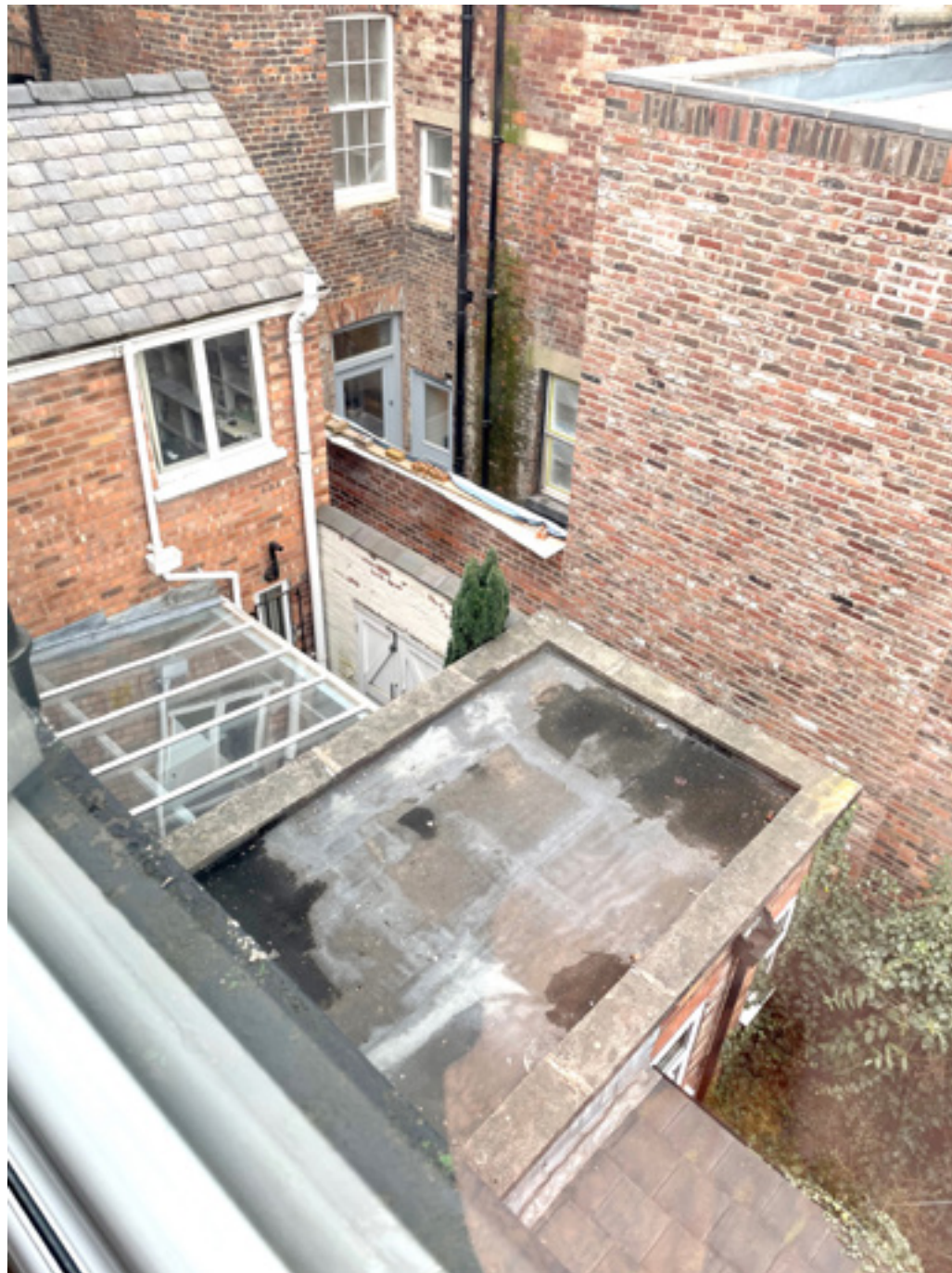
View from the second floor window of 27 Byrom Street Looking at the existing single story flat roof extension to 27 Byrom Street and the pitched roof extension to the rear of 25 Byrom Street
