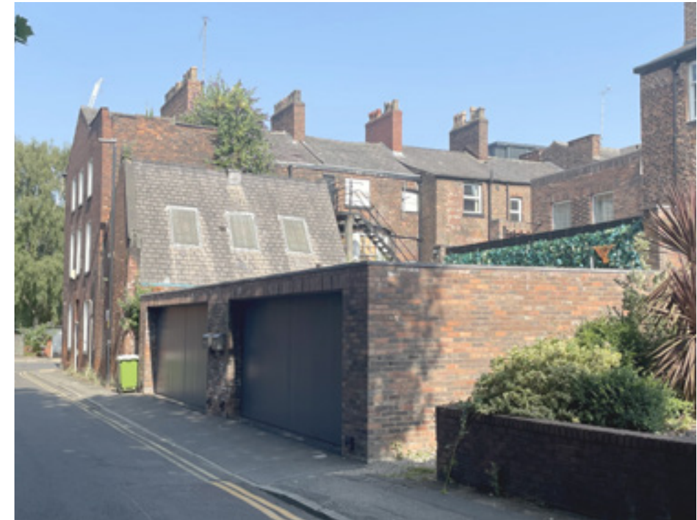
Rear elevation of 27 Byrom Street from Camp Street
