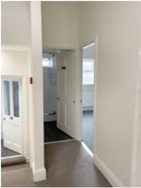
02. View of later additions of a stud wall and shower room
