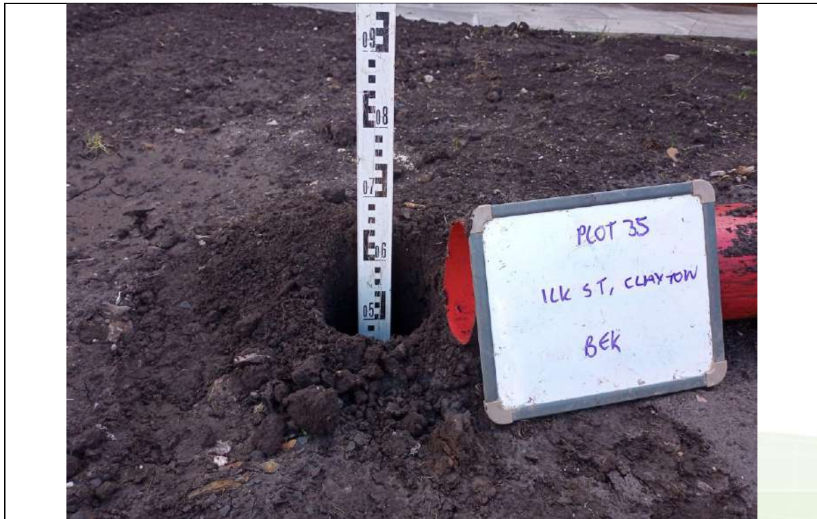
Photograph 1: Validation of Garden Capping Thickness
