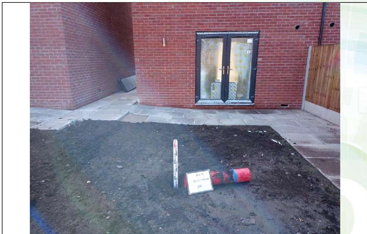
Photograph 2: Validation of Garden Capping Thickness
