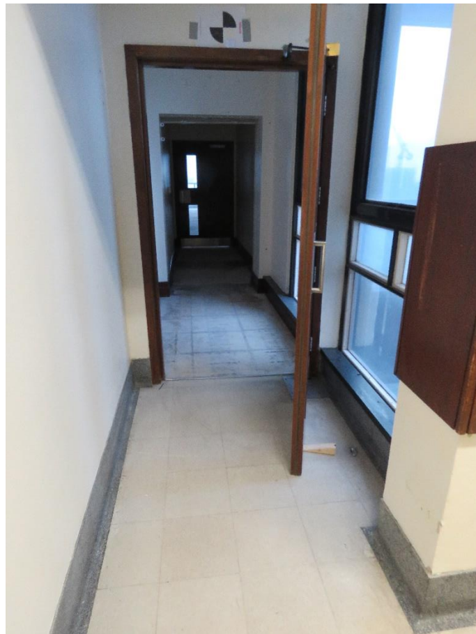
15.11 View north from the eastern stair back through the separating fire lobbies.
