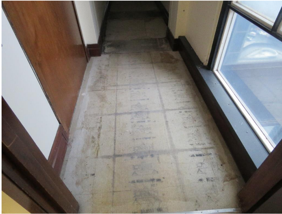
15.12 The removal of later floor coverings has shown that the terrazzo tiles continue from the stair through towards the office space and stop in line with the fire shutter.
