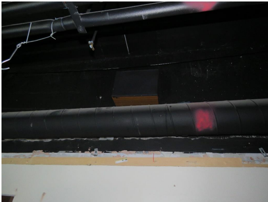
15.03 A speaker within the ceiling void was most probably from an early tannoy system.
