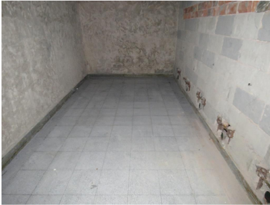
15.14 View of the eastern WC with all cubicles and services removed, the western WC survives in the same condition.
