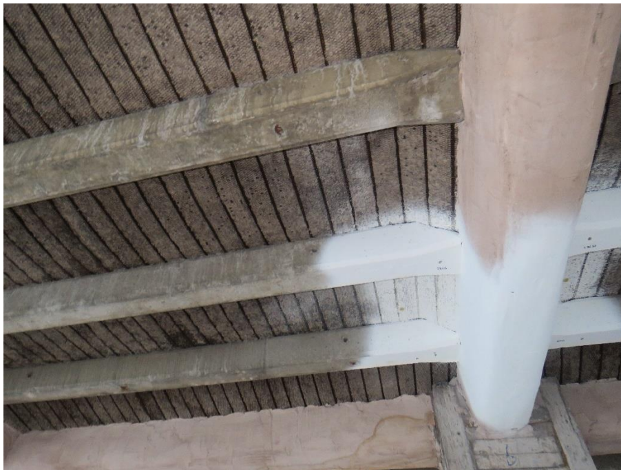
15.07 View of the floor slab construction with retained wire mesh shuttering utilised to the tower floor slabs. Also note that the primary beam was plastered, and a sample intumescent paint application can be seen for the fire protection of the buildings structural concrete.
