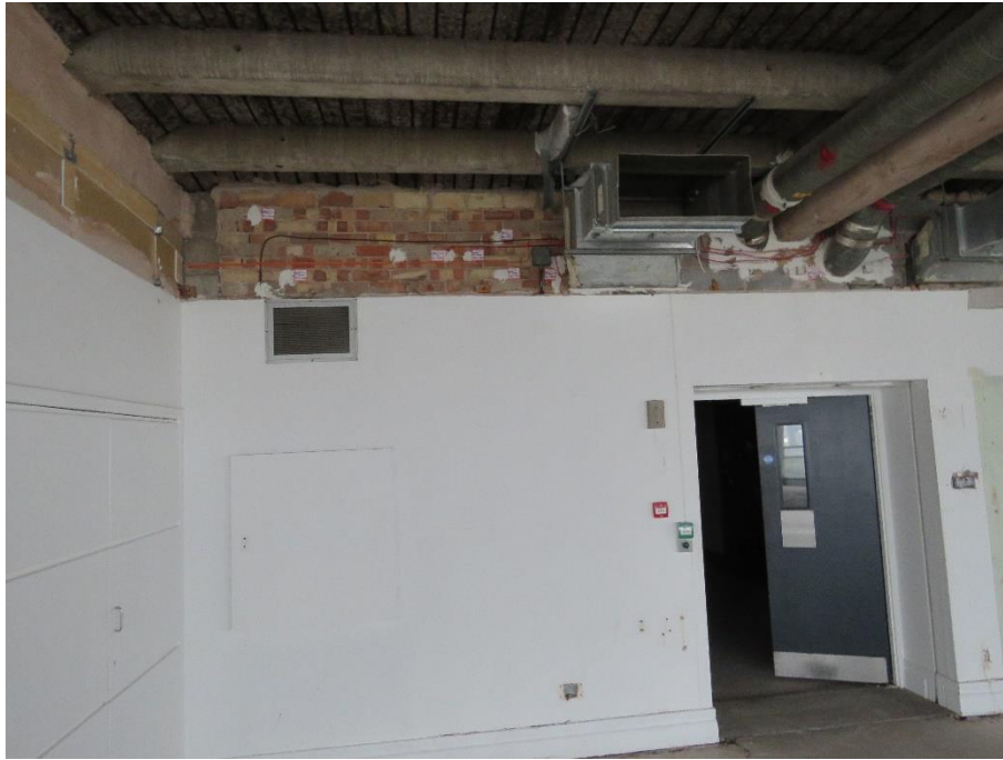
15.06 View towards the lift lobby with services cut back and brick partition.
