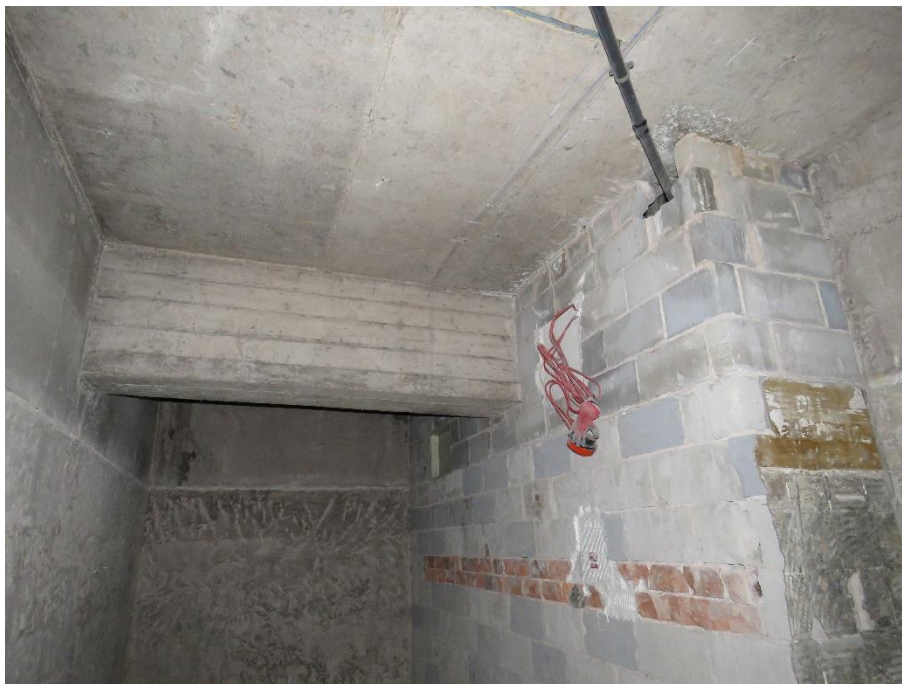
15.15 View of the structural concrete slab of the service core utilising shuttered concrete.
