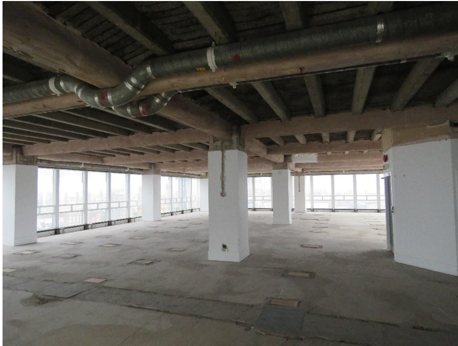
15.04 Looking east across the tower floor plate.
