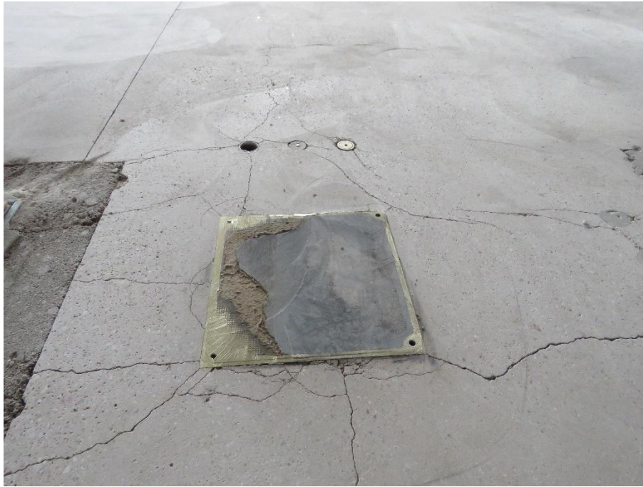
15.08 Detail of a brass floor plate uncovered below the carpet.
