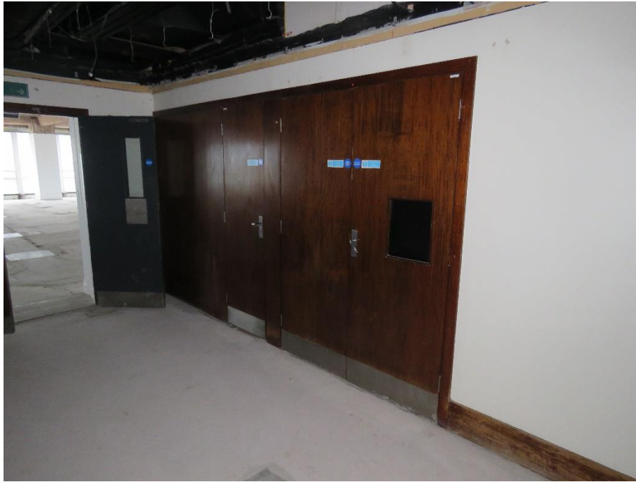
15.02 View of the original riser cupboard doors.
