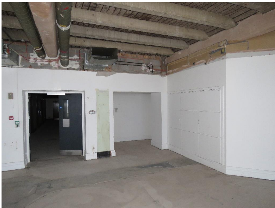
15.05 View toward the Telelift area following strip out of the screen partition and track.
