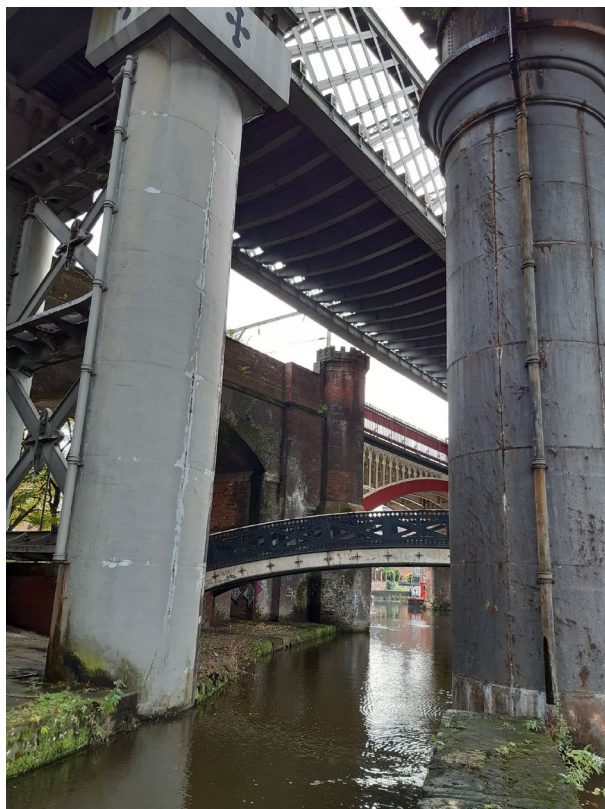
Photographic Plate No. 03: Downspout sampled on right and downspout from tramline on left of photograph
