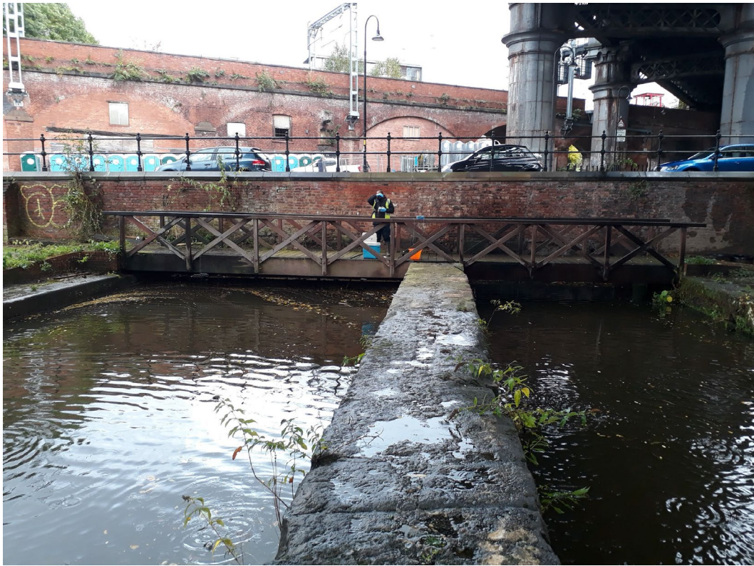
Photographic Plate No. 05: Stone quay within canal basin from downspout looking east
