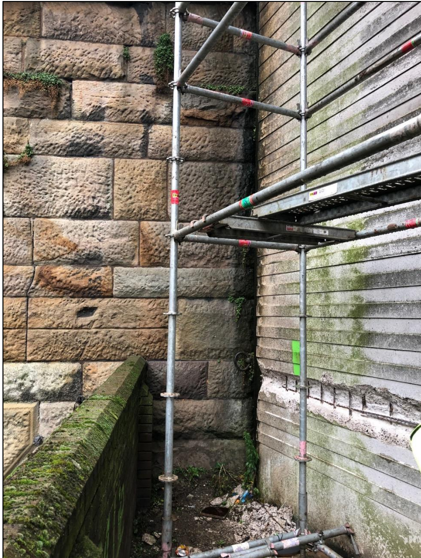
Figure 3.1: Image showing the interface between the existing concrete column and the stone abutments
