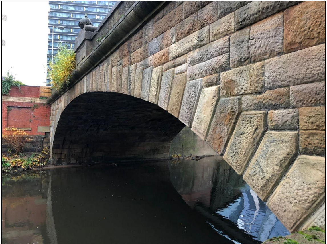
Figure 2.3: View towards the stone abutments of the bridge on the west bank of the River Irwell
