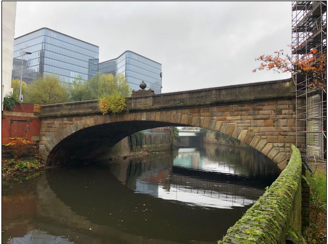
Figure 2.2: View towards the elliptical arch of the southern elevation of Victoria Bridge, looking north west
