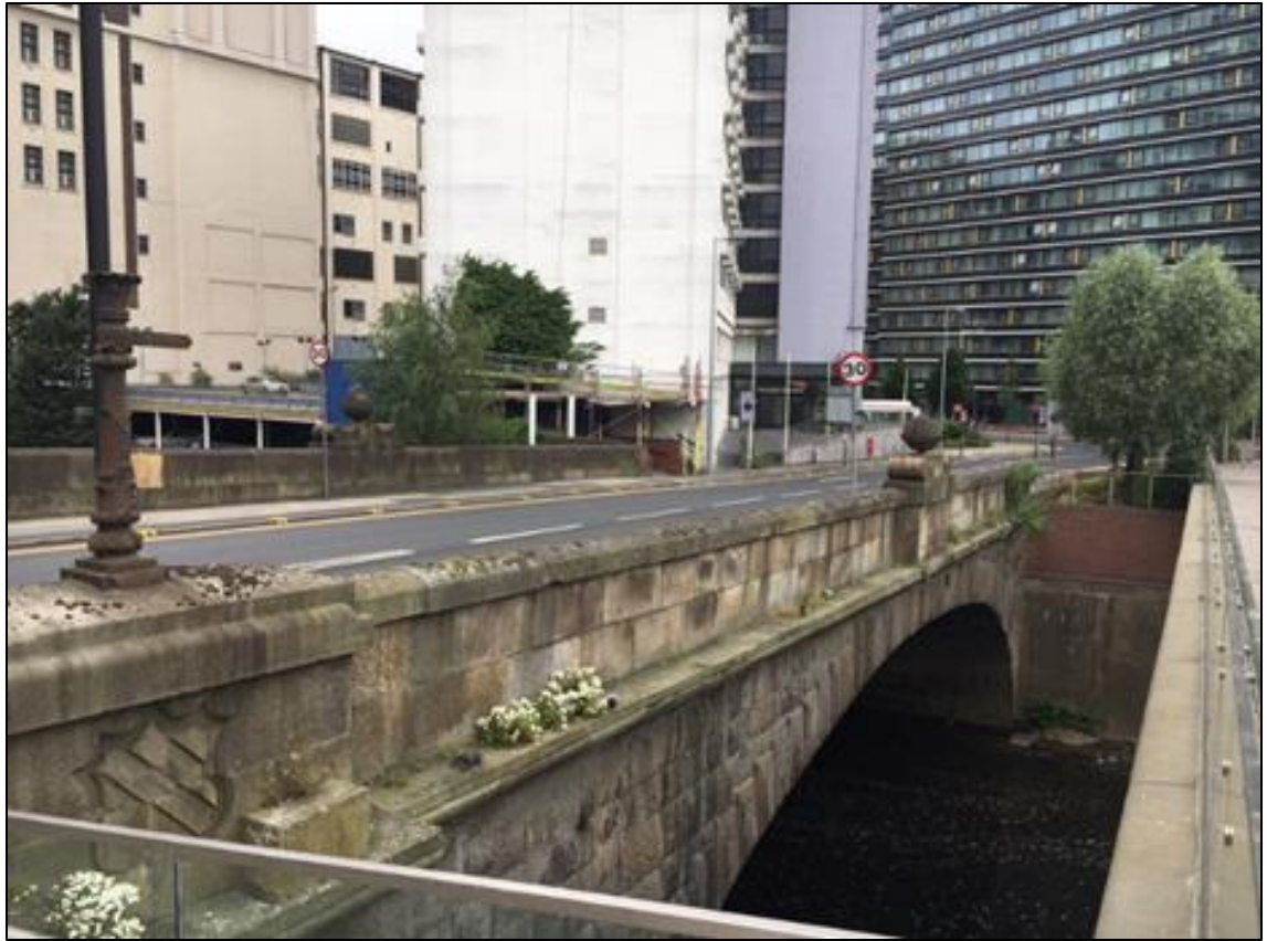
Figure 2.1: View of the north east side of Victoria Bridge from the east bank of the River Irwell
