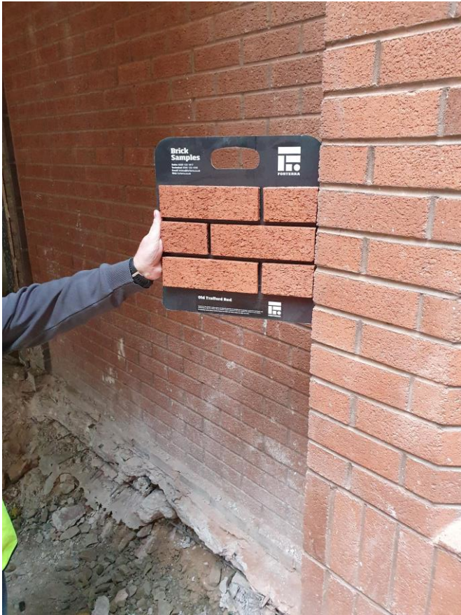
Red brick with buff mortar to match existing – Photo Document
