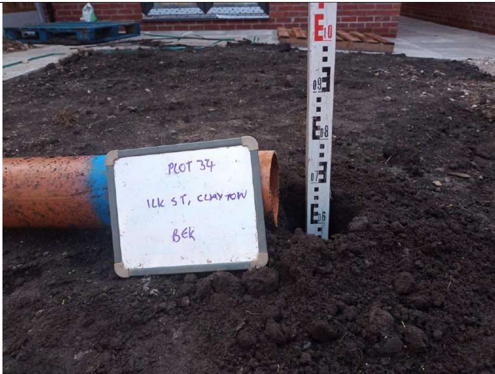
Photograph 1: Validation of Garden Capping Thickness
