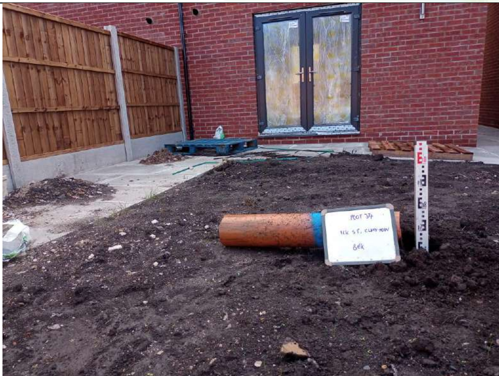
Photograph 2: Validation of Garden Capping Thickness
