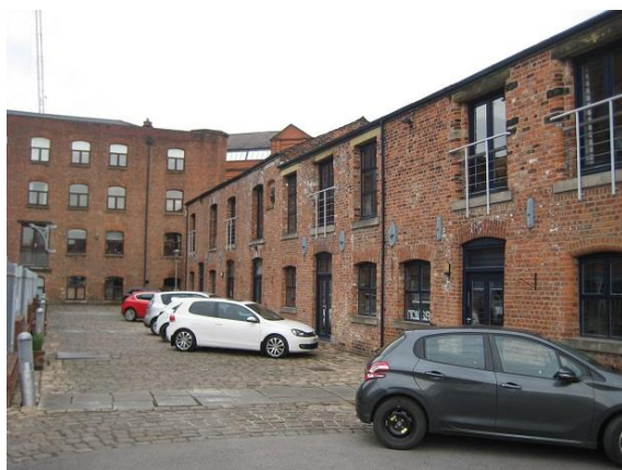
Figure 2.2: Listed Stables Block in foreground. Listed Junction Works Building to rear.
