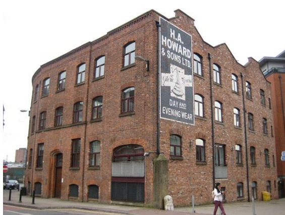
Figure 2.7: Grade II Listed Junction Works
