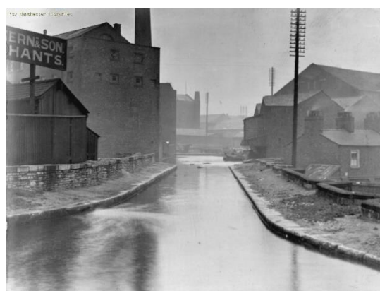
Figure 6.2: 1903 photo looking west. Site to right beyond aqueduct.
