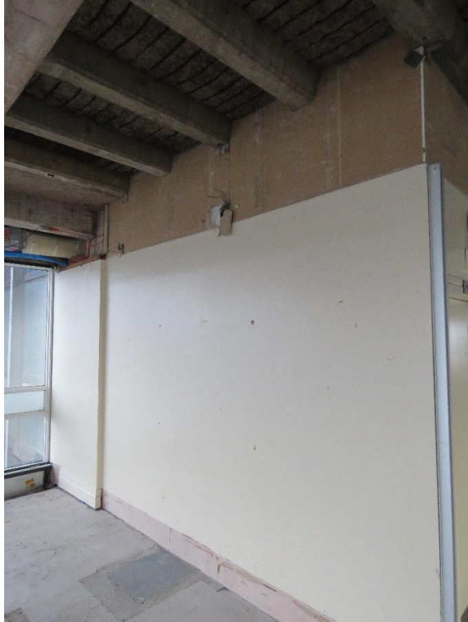
14-04 View of the internal partition between the office space and the stair lobby, being a non-original partition retained at present for fire separation.
