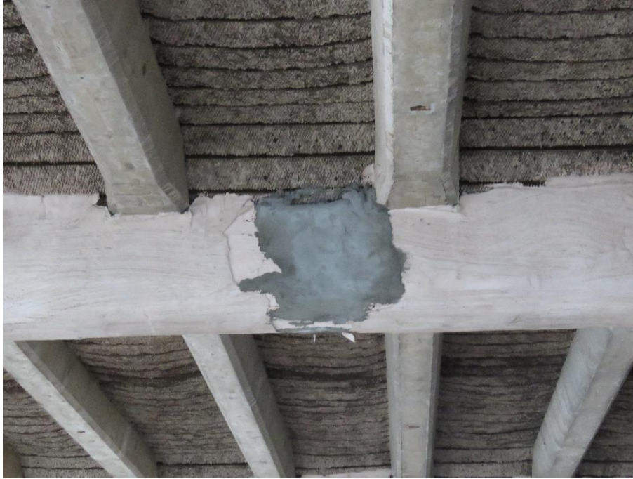
14-02 View of one of the repairs following intrusive investigation of the primary structural concrete beams.
