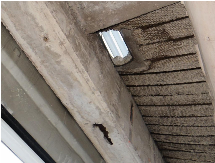
14-03 View of the tower floor slab construction showing the use of a metal mesh as shuttering (compared to tradition timber shuttering used at podium level) that is retained in situ.
