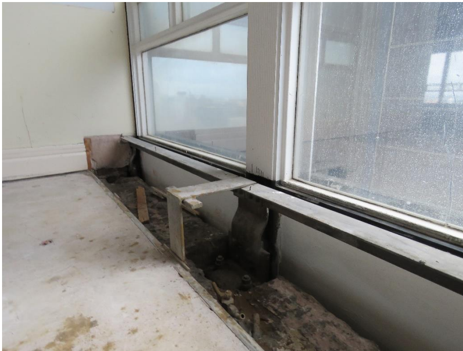
14-01 Close up view of the perimeter structure that housed the Weathermaster heating system.
