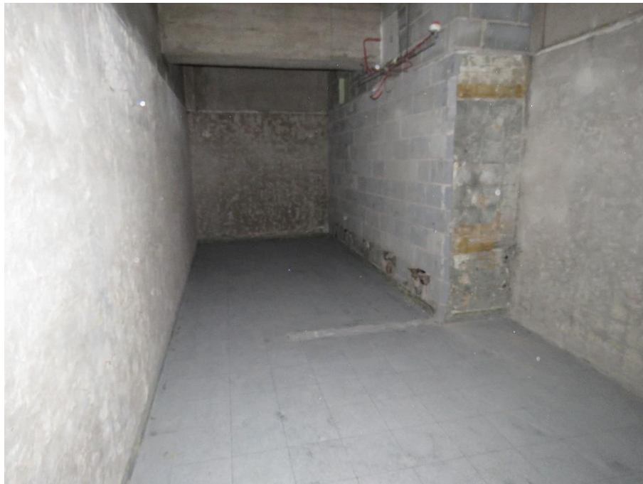
14-05 View of the eastern 14 th floor WC following strip out with terrazzo floor tiles surviving.
