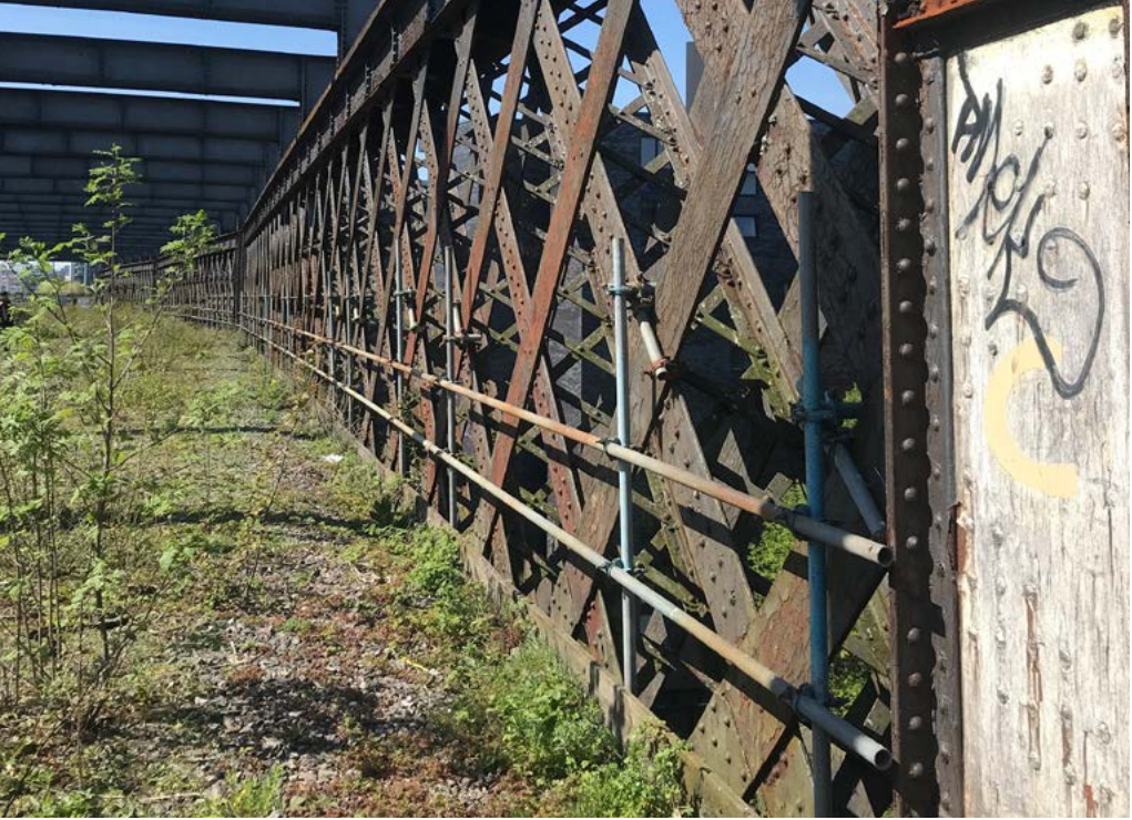
Photo of existing scaffolding poles
