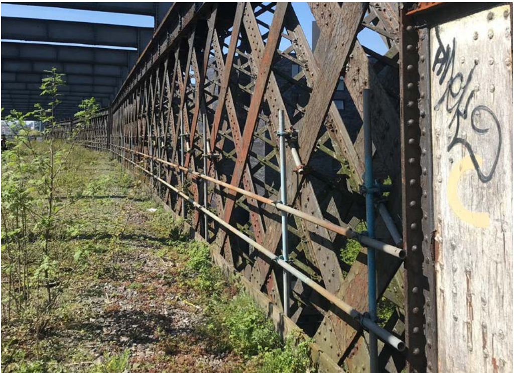
Photo of existing scaffolding poles
