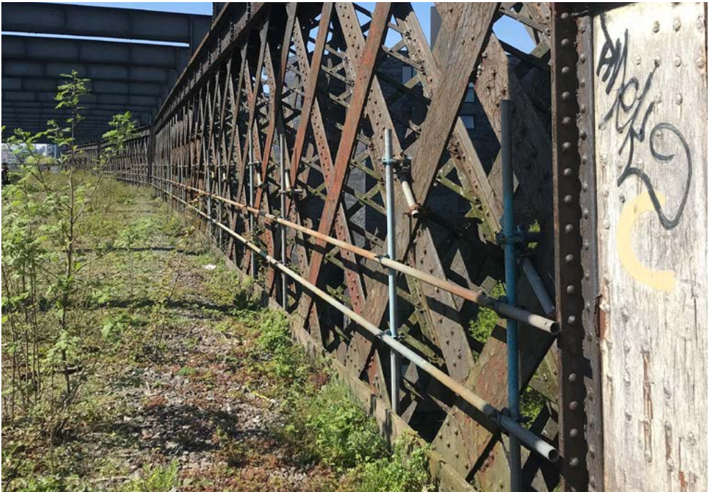
Photo of existing scaffolding poles
