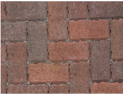
Car parking spaces finishes with Marshall's Piora permeable paving in Brindle colour to parking spaces and Buff colour to 1.2m wide safe pedestrian route
