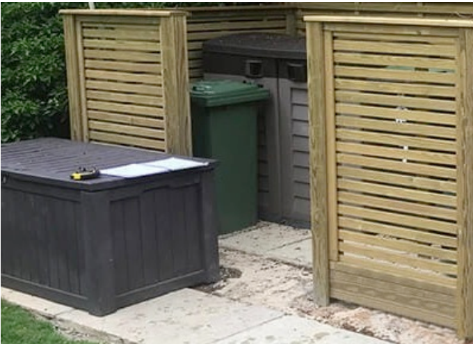
1.2m High timber fencing to open refuse store area in front garden
