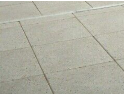
New paving to be Marshall's Perfecta 450x450mm concrete paviors with a Natural colour finish
