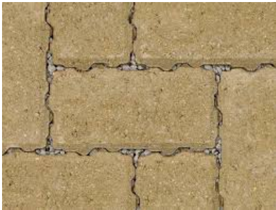
Car parking spaces finishes with Marshall's Piora permeable paving in Brindle colour to parking spaces and Buff colour to 1.2m wide safe pedestrian route
