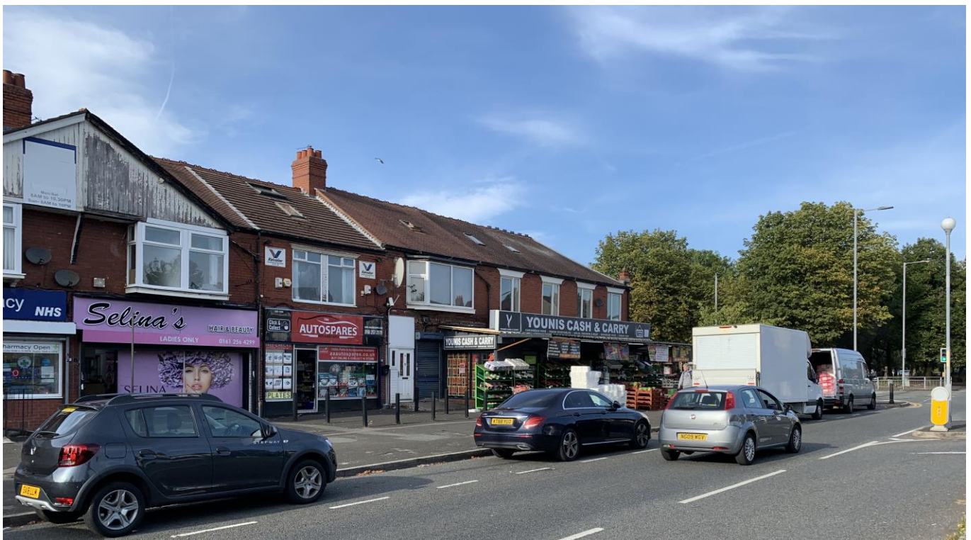
Photograph 1 Application site as viewed from Kingsway
