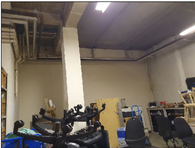
Photo 8 Example of the basement rooms
