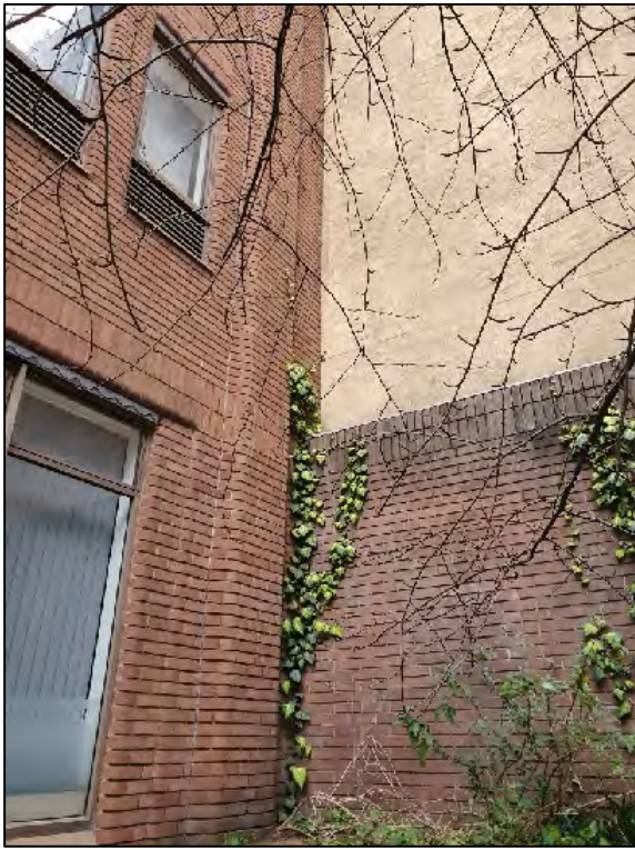
Photo 1 Small compartment of vegetation at the foot of the structure at the paved eastern frontage
