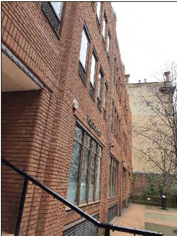
Photo 3 The red brick aspect of the structure
