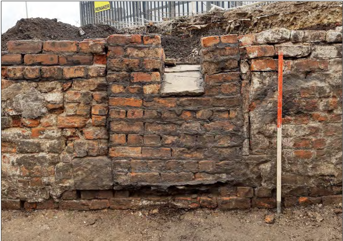
Plate 23: The blocked-up doorway and coal chute 1008 associated with House 1, looking south-east
