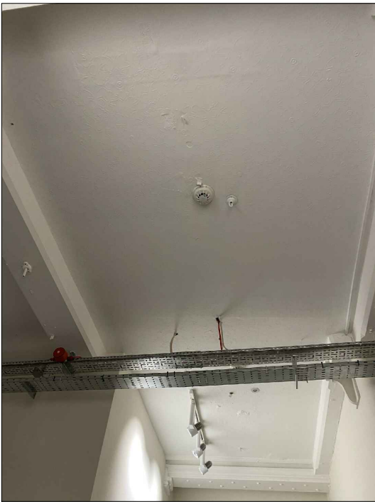
LINCRUSTA CEILING / TIMBER / STEEL BEAM
