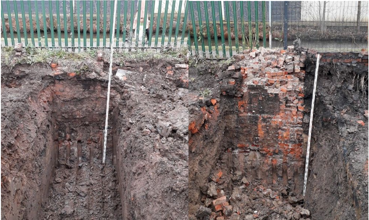
Examples of 'hit & miss' grubbing out to natural soils along site boundary adjacent to canal during Mobilisation 1.
