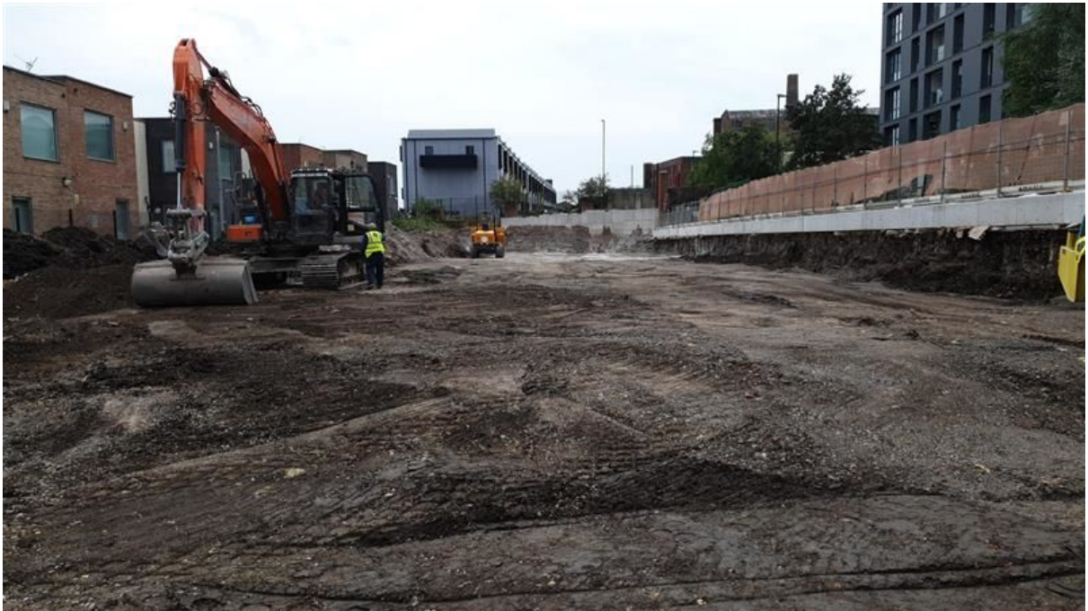
Forming site levels for permanent piling mat during Mobilisation 2.
