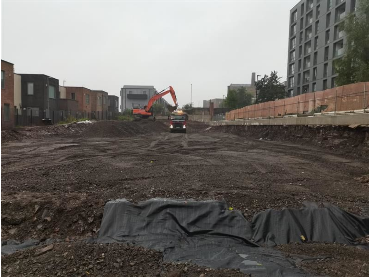
Trimming and compacting surfaces. Disposal of surplus materials.
