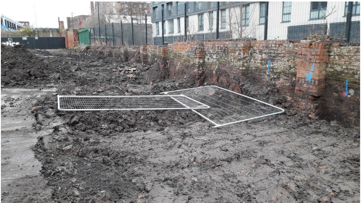
Example of grubbing out along canal side.
