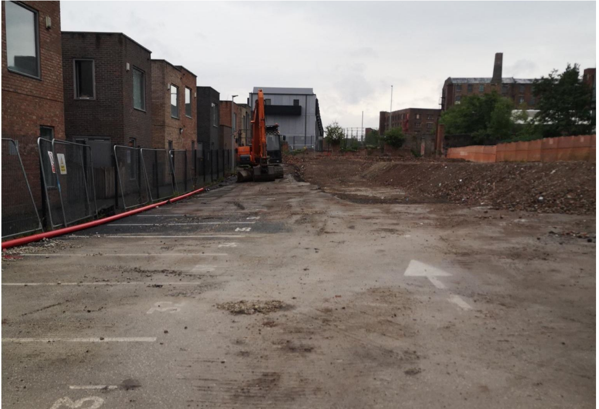
Forming temporary works piling mat for contig pile retaining wall during Mobilisation 1.
