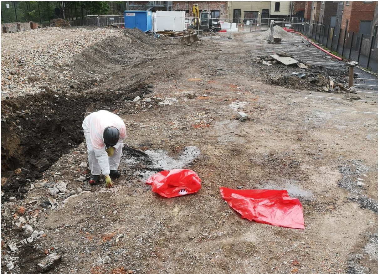
Localised hand picking of ACM by specialist.
