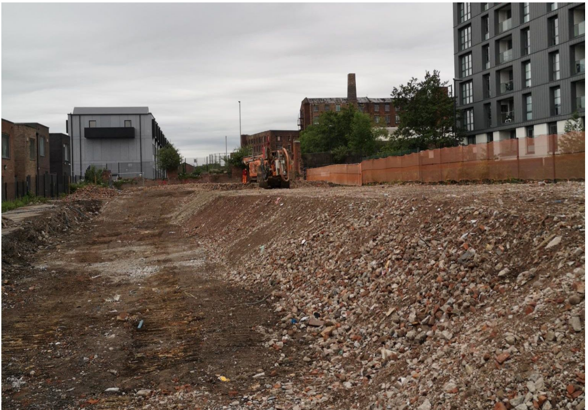
Forming temporary works piling mat for contig pile retaining wall during Mobilisation 1.
