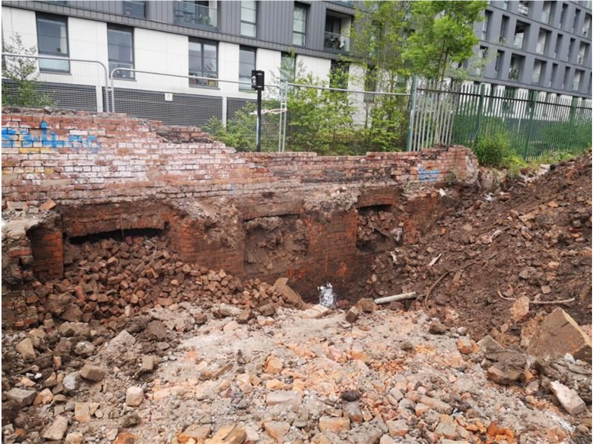
Example of grubbing out along canal side showing relict in-ground structures.
