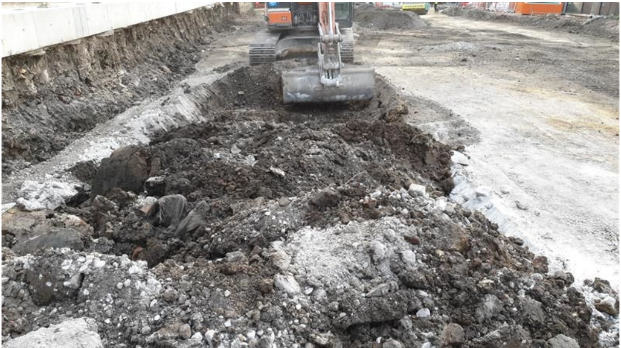
Digging out and re-engineering soft spots.
