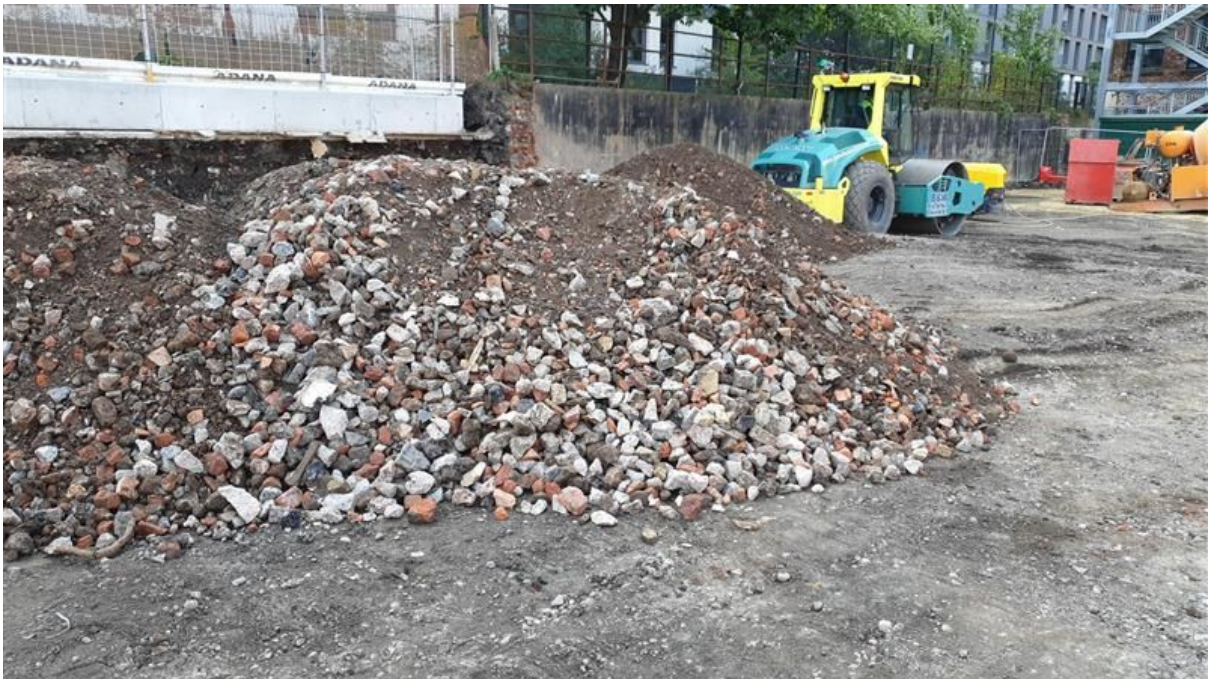
Example of site generated aggregates.
