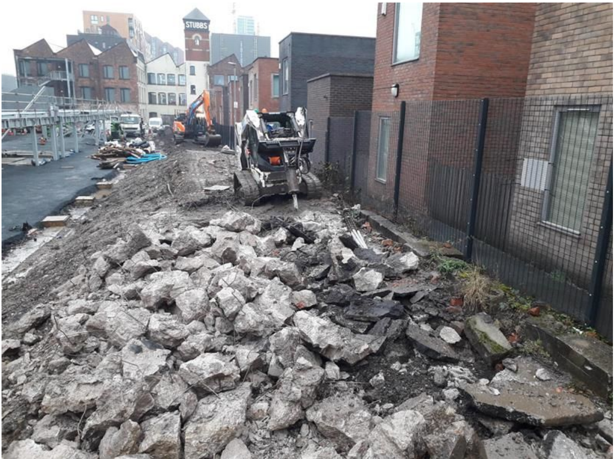
Removal of small area of concrete and retaining soil 'berm' during Mobilisation 3.
