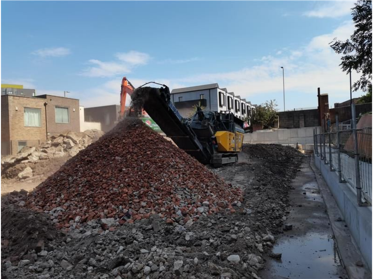
Site generated aggregates from relict structures used to form pile mats.
