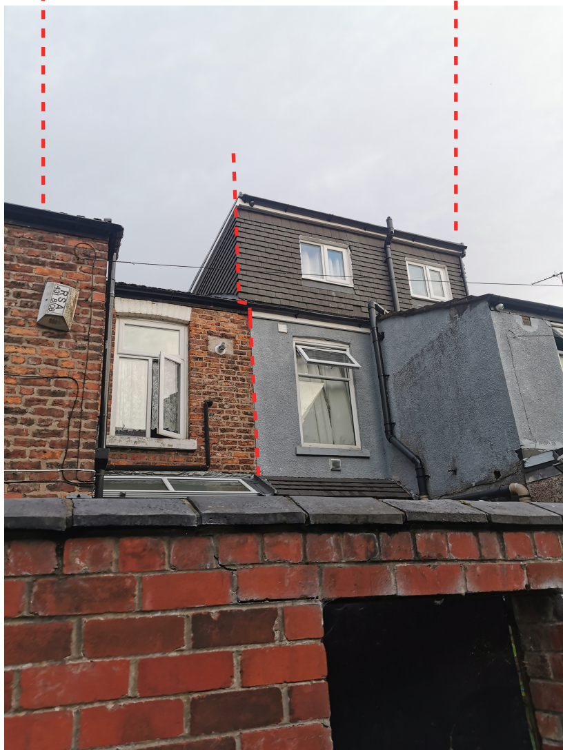
Rear of No 16 ( existing dormer)
