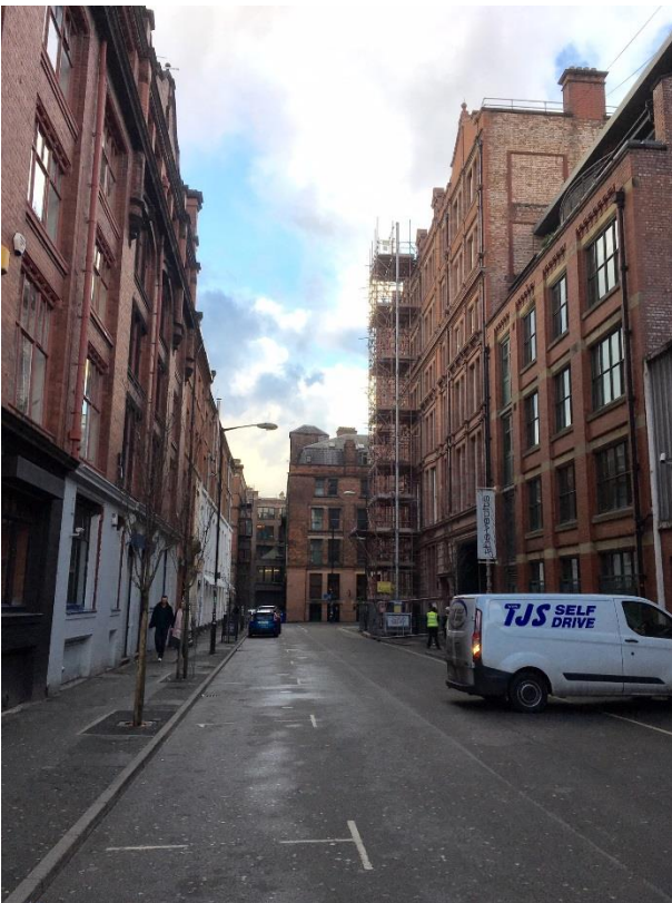
Fig. 19: View towards the site from Tariff Street
