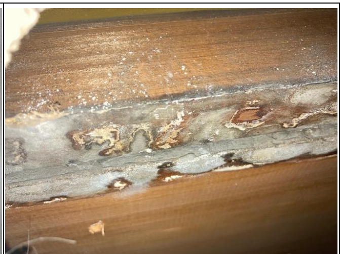
Materials of 1960s Ceiling
