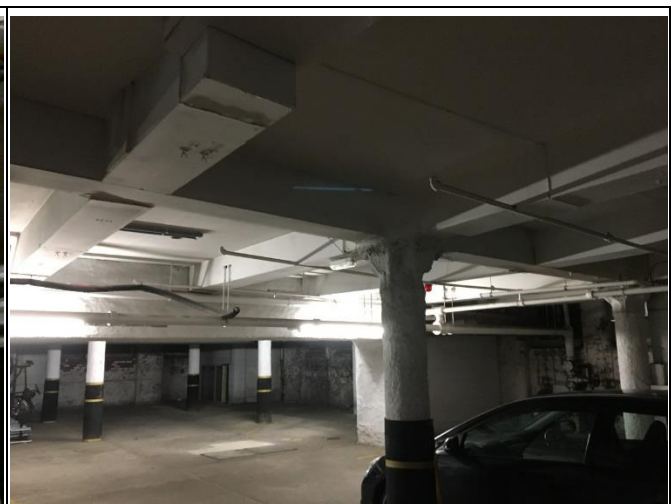
Garage with Columns and Beams
