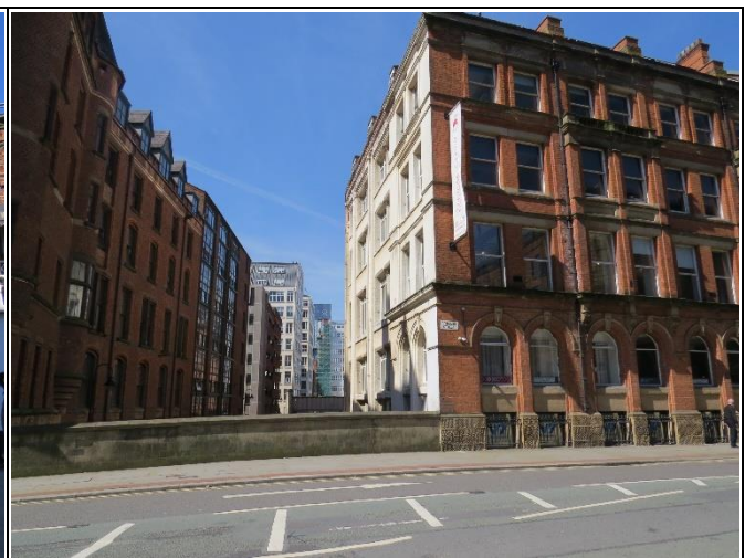
Bridge over Rochdale Canal
