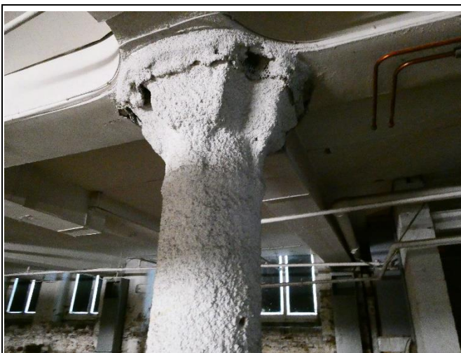
Garage Area with Rendered Pillar (Fire-proofing)
