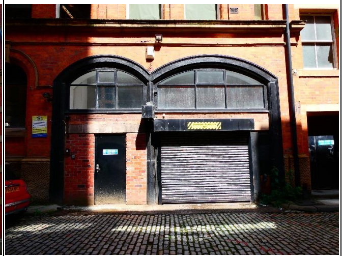
Former Loading Bay with Altered Openings
