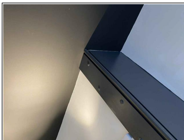
Existing Perimeter Bulkhead of Street Entrance
