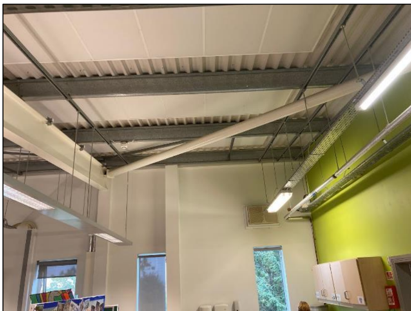
Photograph 9 showing the interior of the building
