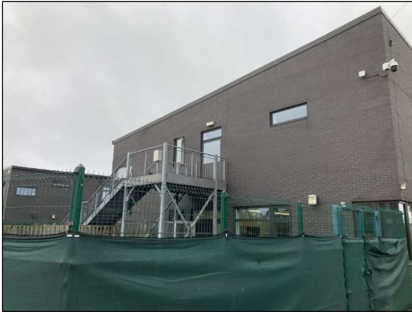
Photograph 7 showing the external masonry
