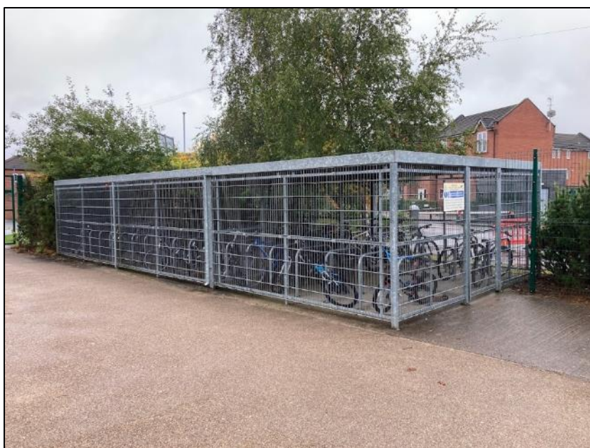
Photograph 5 showing the bike shelter on site
