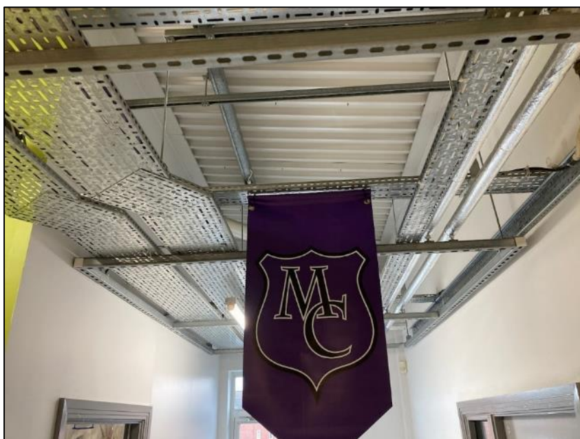
Photograph 10 showing the interior of the building
