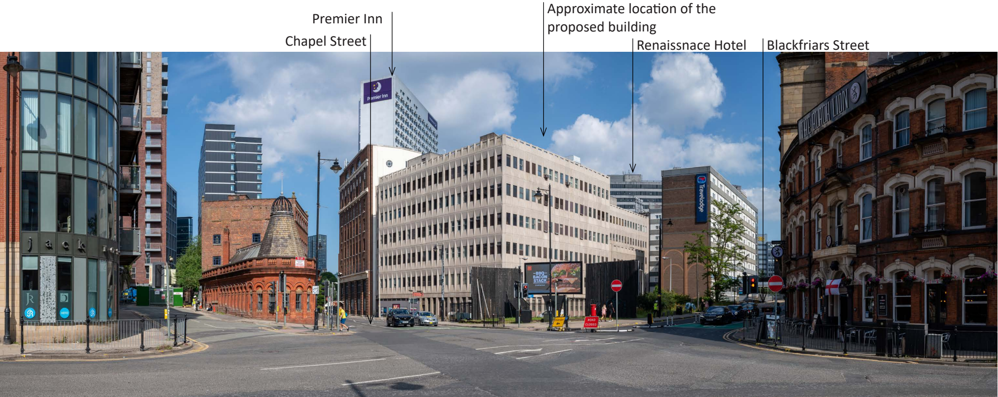
Photograph 8.2 - View from Backfriars Bridge and Chapel St, looking east towards the site
