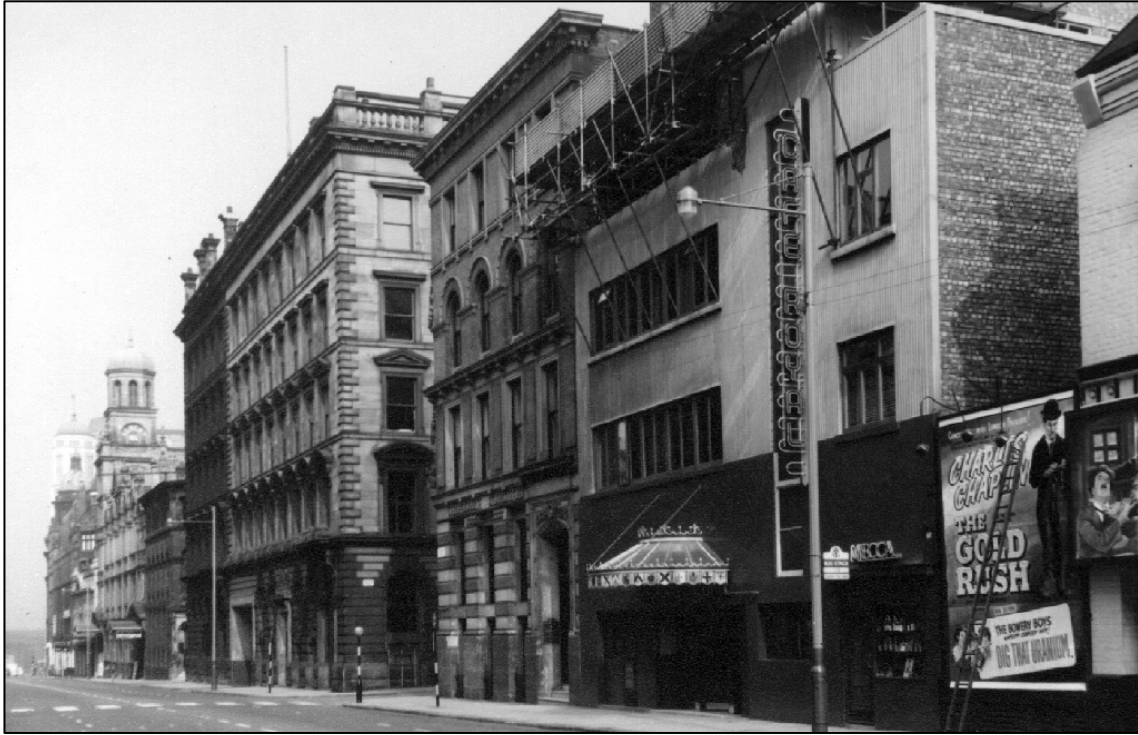
1956: Photograph showing No. 47 Peter Street at the centre of the image, before the alterations of c. 1963.
