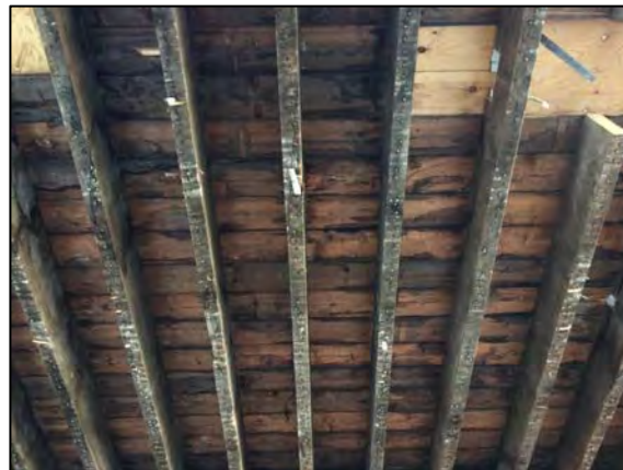
Detail 22: Typical ceiling arrangement at second floor level with marks for former lath and plater visible where removed.
