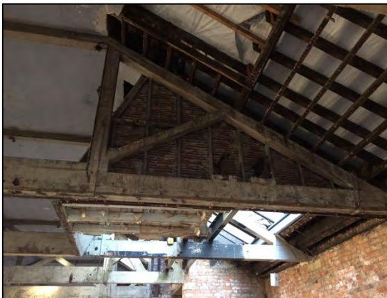
Detail 13: Rear of original timber lath and lime plaster enclosure to roof light above hoist.
