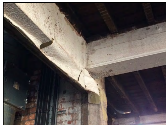
Detail 42: Truncated chamfer and stop detail at edge of secondary hoist enclosure confirming this is a later addition.
