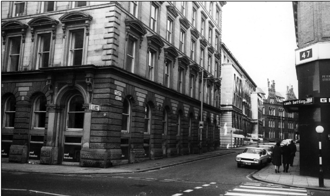
1973: Photograph showing Southmill Street with No. 47 Peter Street to the extreme right-hand side of the image. The alterations to the ground floor of c. 1963 are visible however the Building Society has been replaced by a bookmakers. (Manchester City Archives)
