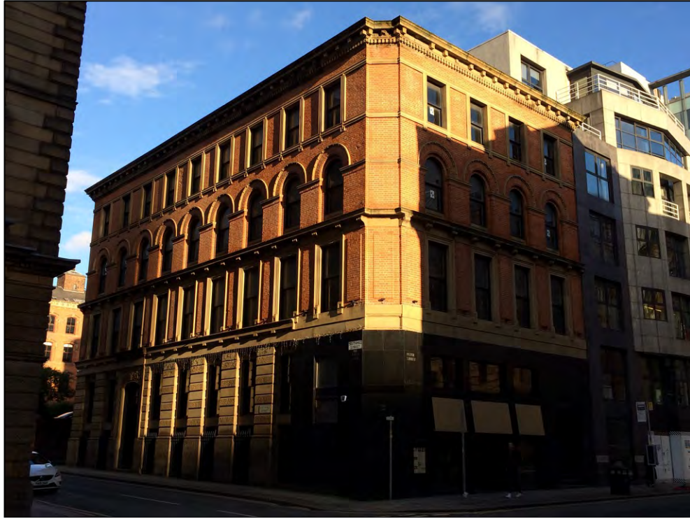
Plate 4: Oblique view of Southmill Street and Peter Street elevations
