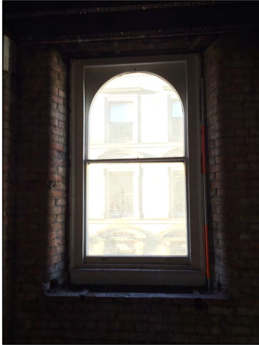
Detail 27: Typical one-over-one sliding sash window to second floor level with round-headed upper sash to match external opening.
