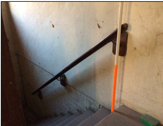
Detail 37: Surviving section of outer wall handrail to ground floor level of staircase, with wrought iron attachments to staircase enclosure wall.
