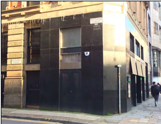
Detail 5: Polished black marble shop front to the Peter Street / Southmill Street corner, constructed in 1963 for the Temperance Permanent Building Society
