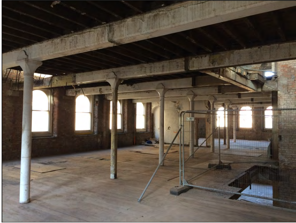
Plate 10: Oblique view of the second floor with the central row of cast iron columns
