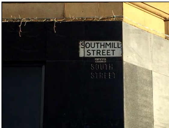
Detail 7: Incised street name "SOUTH STREET" to black marble shop front of c. 1963. Later signage above marks the change in name to Southmill Street in the following decade.
