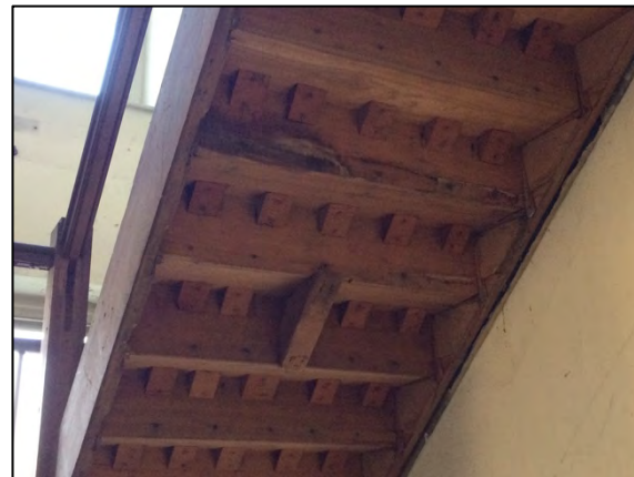
Detail 34: Typical view of the soffit of the c. 1950s timber replacement staircase showing the very high quality of construction to the treads and risers.
