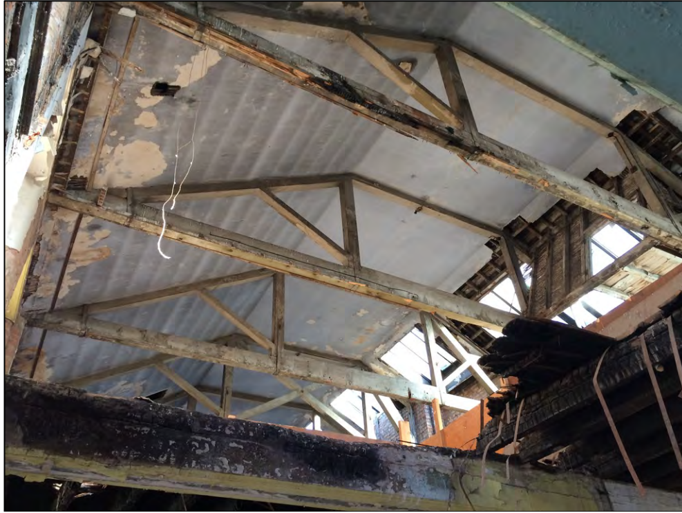
Plate 6: Oblique view of Queen Post truss arrangement to principal roof trusses
