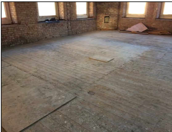
Detail 21: Typical floor board arrangement to third floor level, with later infill following removal of 1896 staircase.
