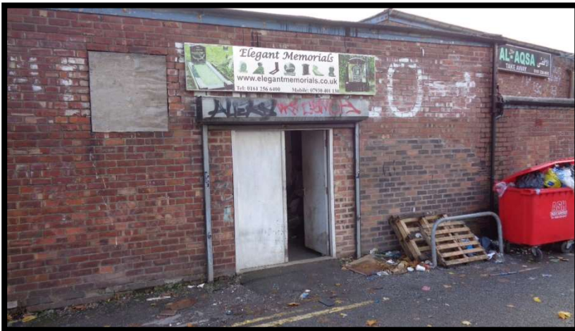
Service access into application property from Brook Terrace
