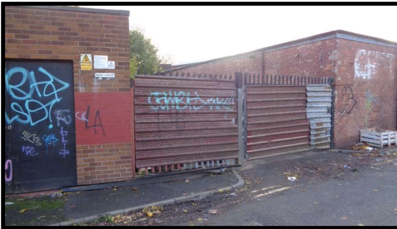
Gates on Brook Terrace to application site service yard
