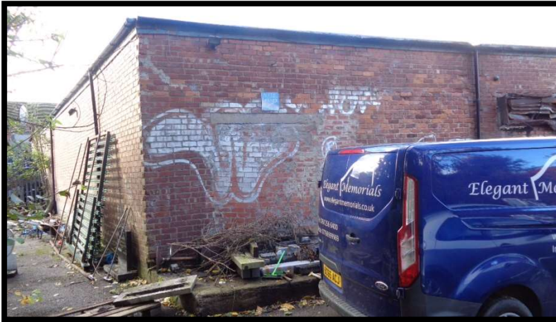
Rear service yard of application property
