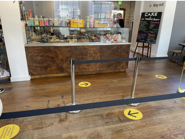
View of the servery, the face of which is to be refinished.
