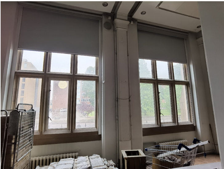
View towards location of the proposed entrance lobby (by others)
