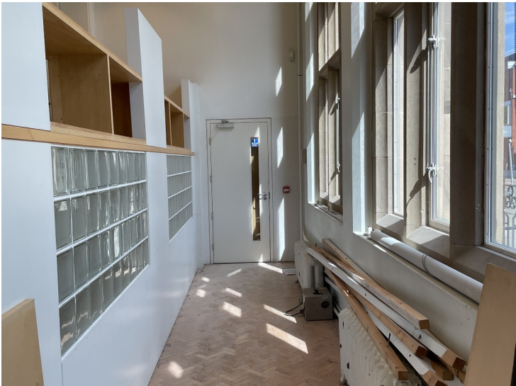
View down corridor between partition wall and Oxford Road facade looking towards Main Hall
