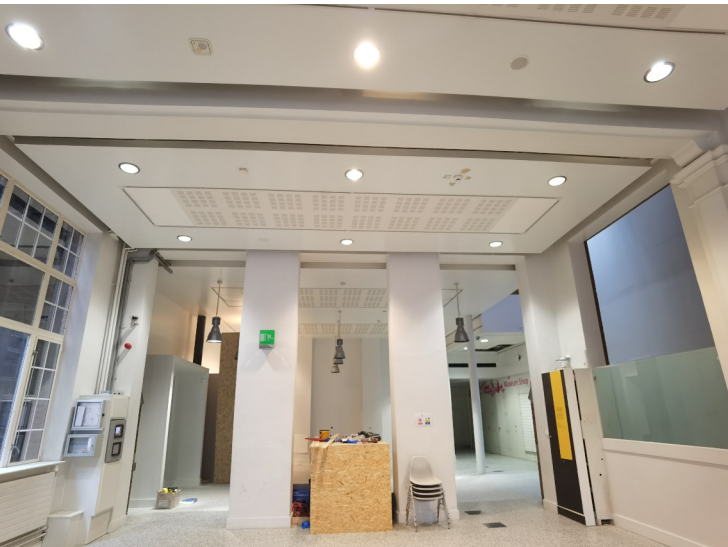
View looking west towards back of the Hall
