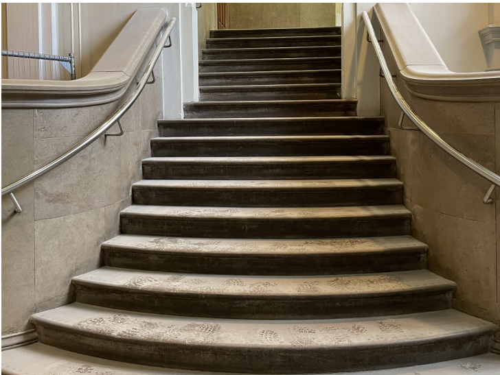
View from bottom of Main Stair
