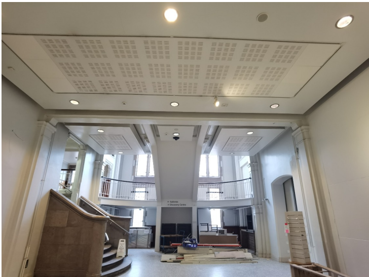
View looking east towards main stair and Shop entrance
