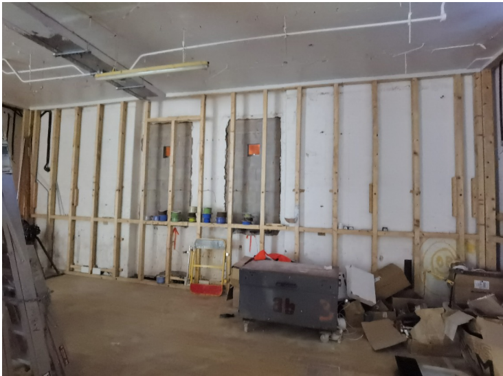
View of north elevation
