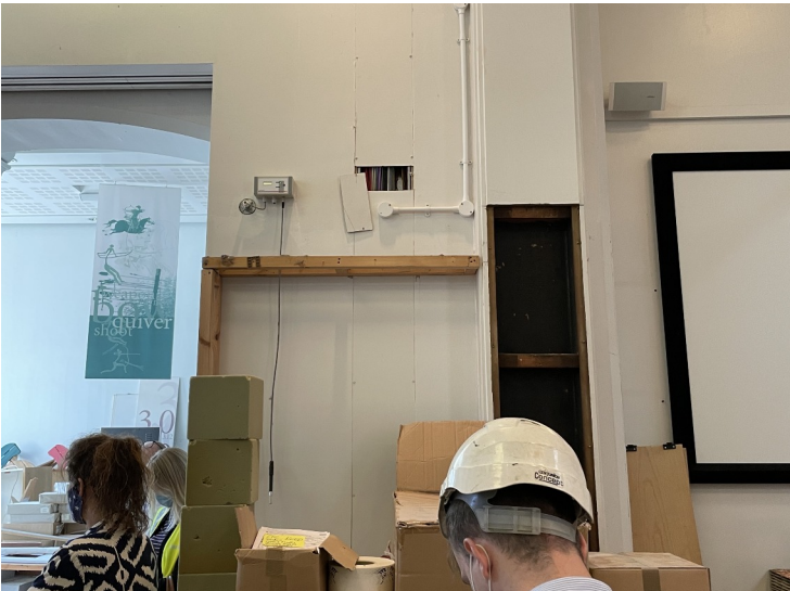
View looking south towards partition between Shop and Entrance
