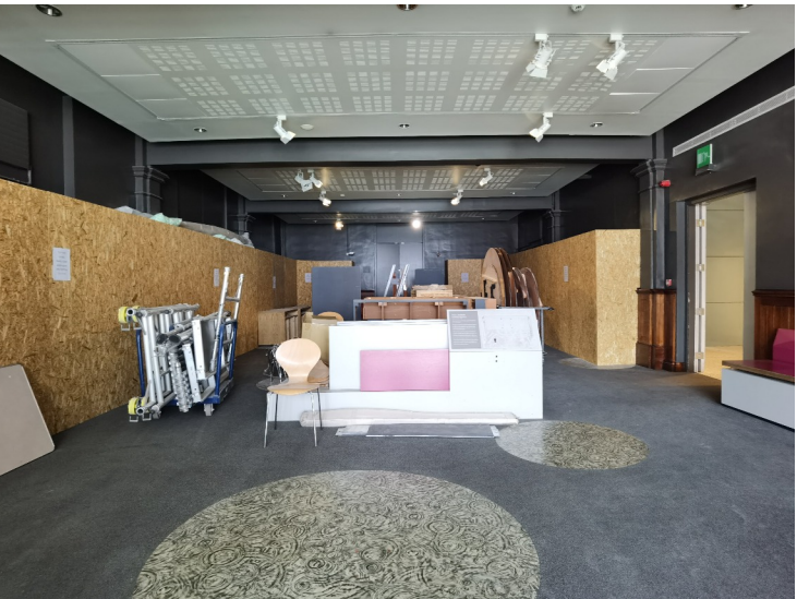
View from top of main stair looking west towards route through to new extension
