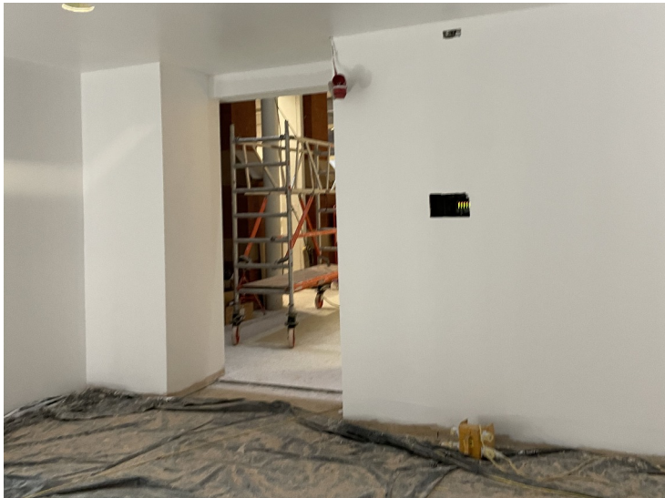
View from circulation space into the Main Hall
