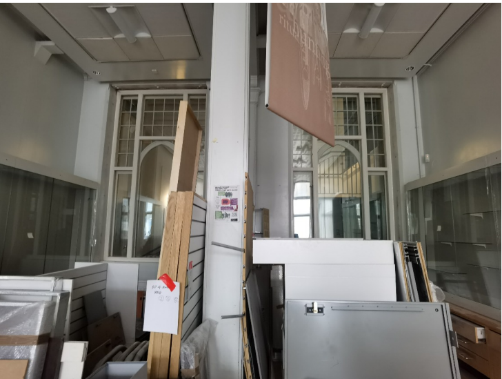
View of partial western facade
