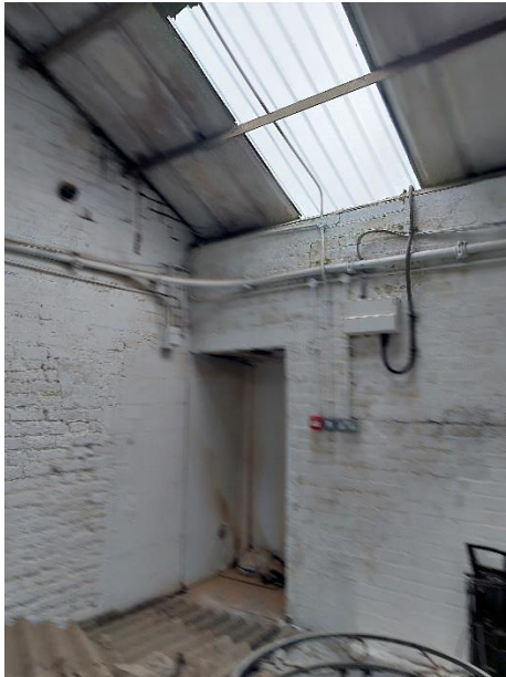
Photograph 3 – Access door connecting to adjacent building.
