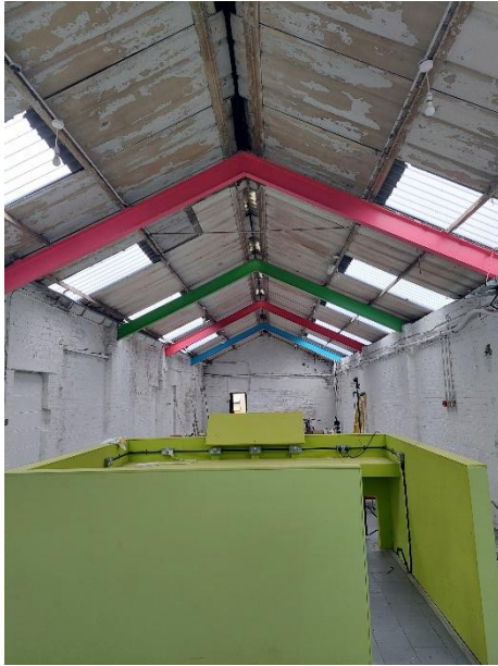
Photograph 1 – Internal view of the upper floor of the building.
