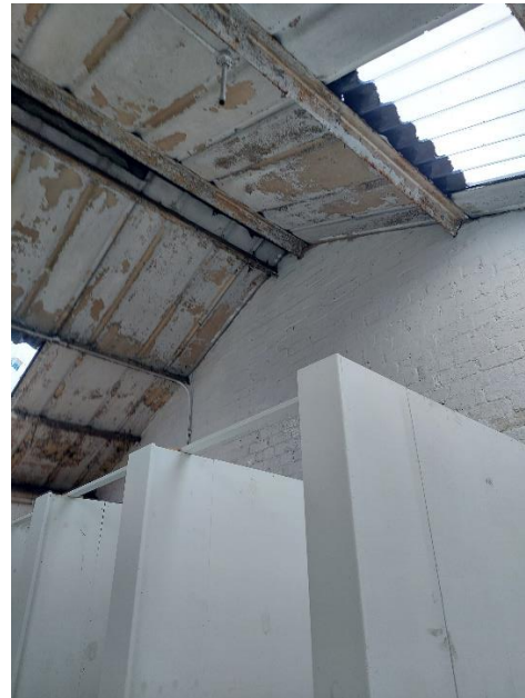
Photograph 4 – Rear of building.
