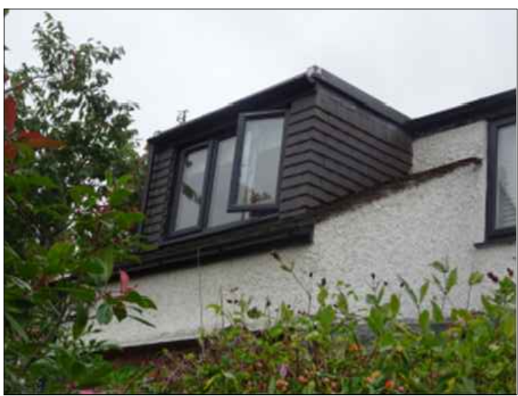
Photograph of Rear Elevation to Dormer of No. 11
