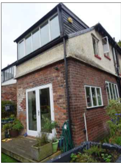
Photograph of Existing Side/Rear Elevation
