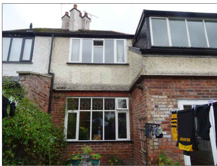
Photograph of Existing Rear Elevation
