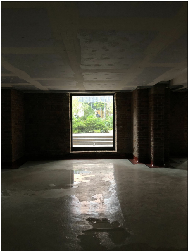
INTERIOR VIEW TOWARDS COURTYARD
