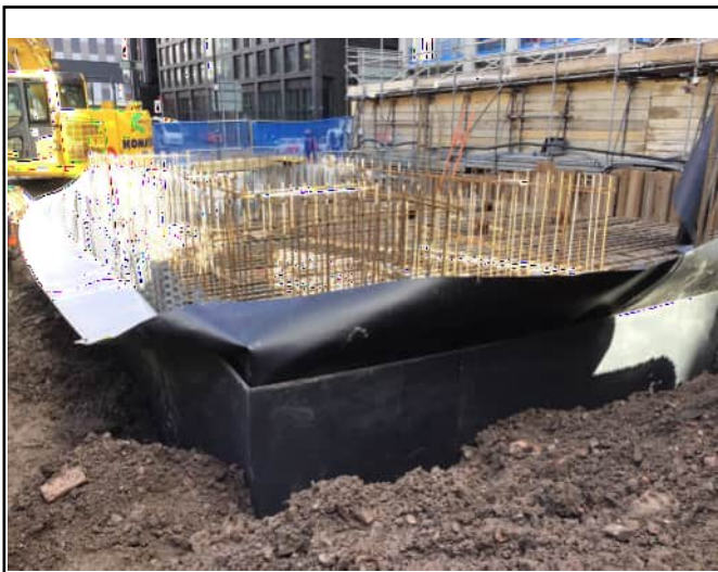
Protection board to base of crane
