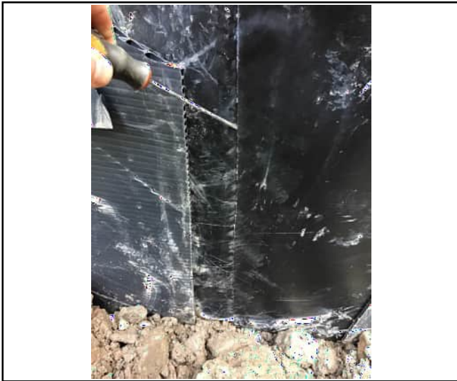
Pick and probe on hot weld before
