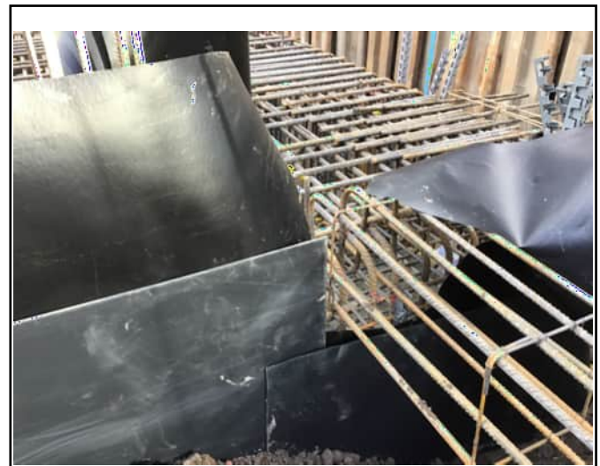
Membrane cut around ring beam
