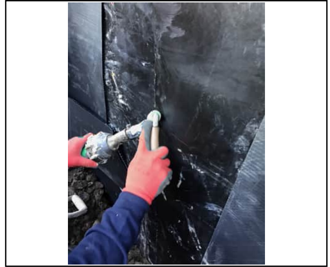
Hot weld in before extrusion
