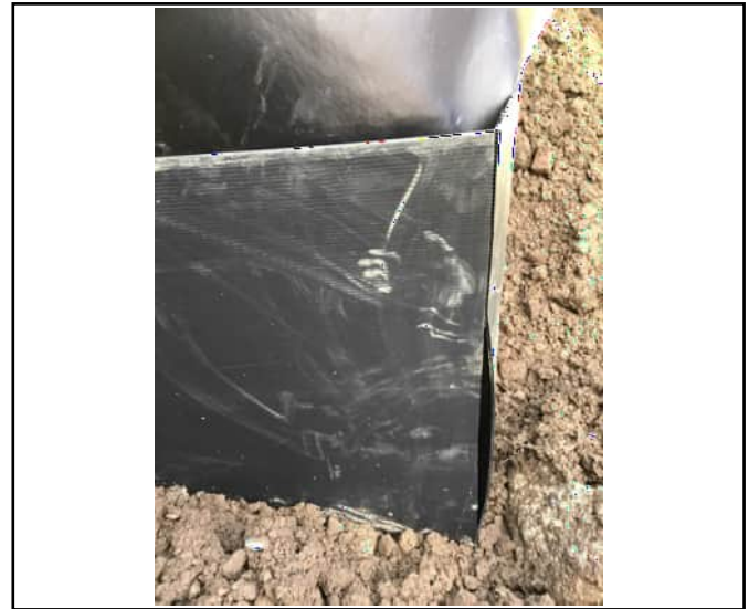
Protection board applied to
