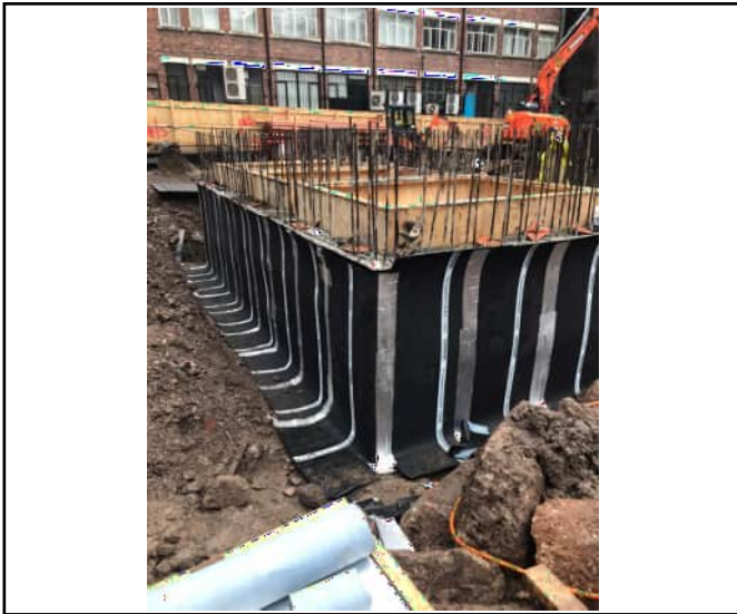
Core protected with protective boarding
