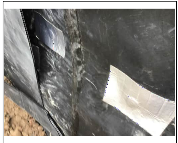
Pegs installed either side of
