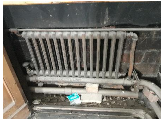
Figure 6 A sectional radiator
