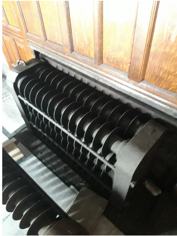
Figure 3 A coil radiator
