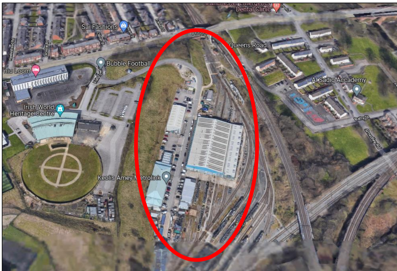
Figure 1: Aerial view of the Queens Road Metrolink Depot.
