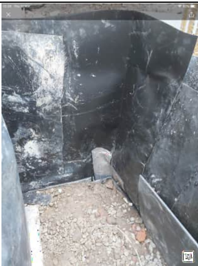
Exterior corner detail of Visqueen
