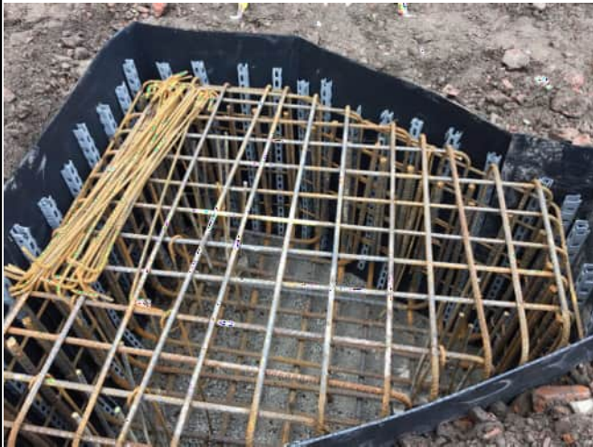
One of the pile caps did not need
