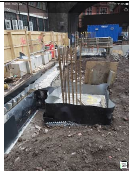
Pile cap and ring beam, both have
