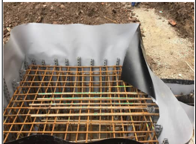
Pile cap with Visqueen Geoseal
