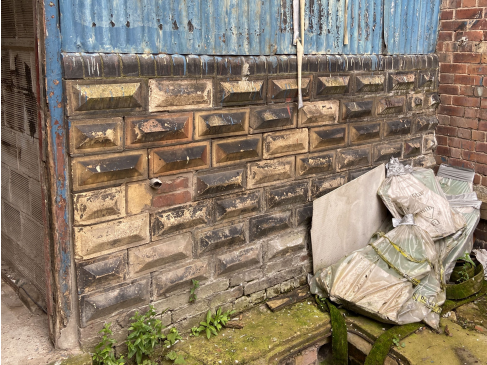
PHOTO OF RUSTICATED TERRACOTTA BLOCKS TO BE RETAINED
