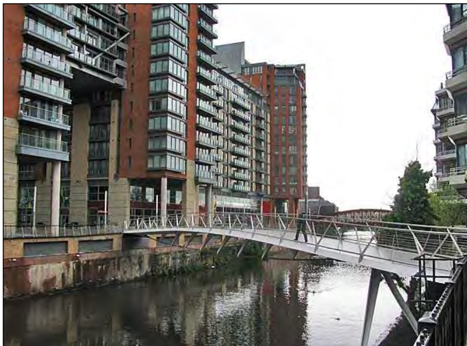
Figure 5.1 Irwell Pedestrian Footbridge
